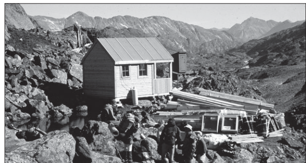
Warm-up shelter construction at the Summit
