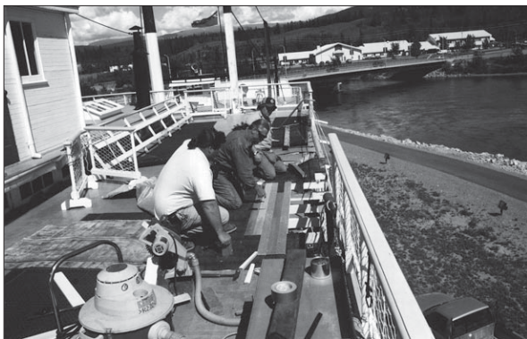
Repairing rotten decking before recanvassing
