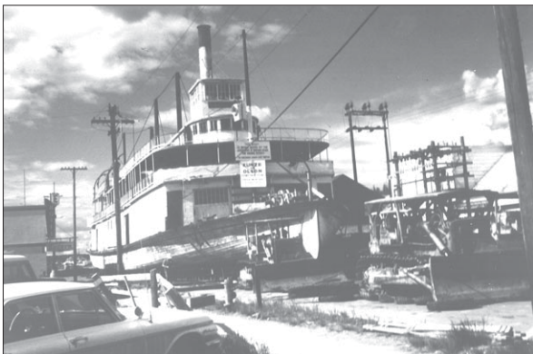
Bulldozers move the S.S. Klondike from the Whitehorse shipyards to its present location, 1966 (G.I. Cameron Collection)
