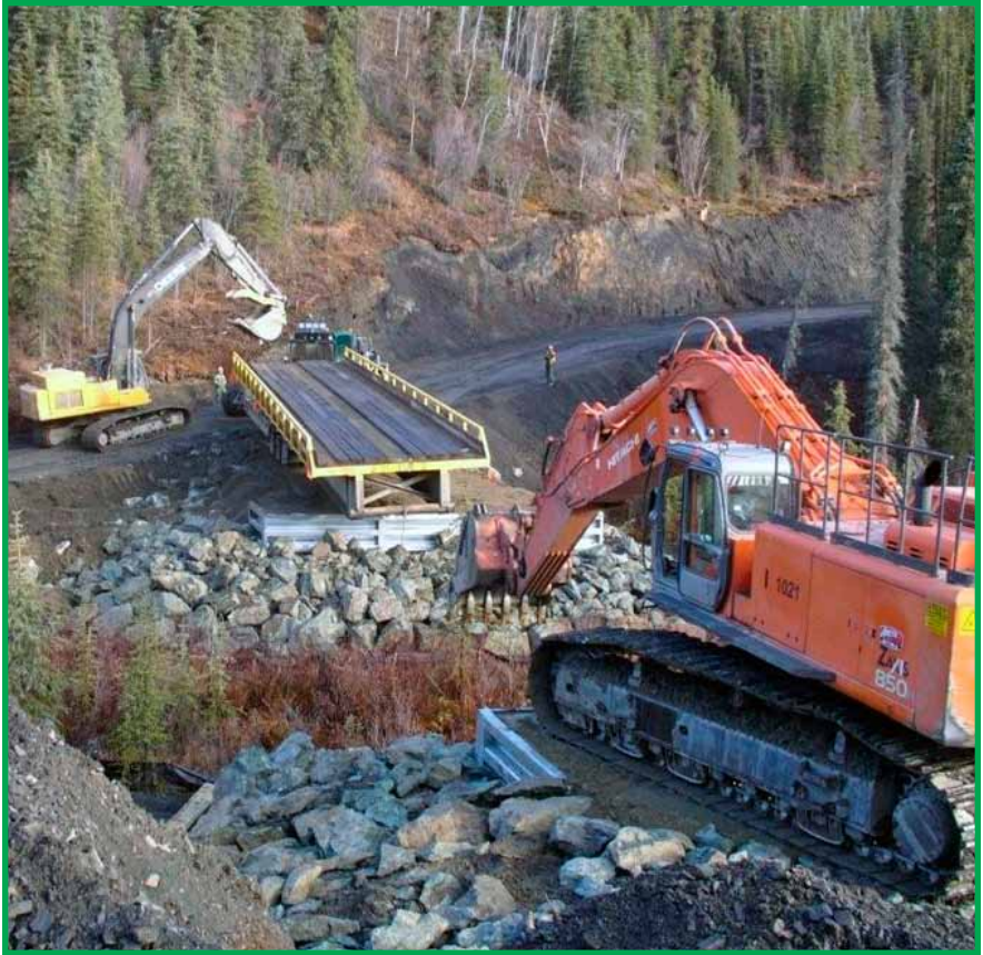
Equipment for this construction project is operated from above the stream bank. Note erosion control measures, silt fences lower left, in riparian zone.
