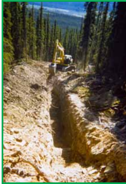
Trench dug using a back hoe. Note top soil and substrate material should be piled a safe distance to the side of the trench.
