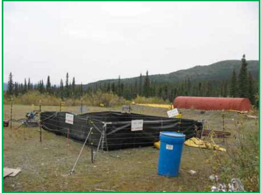
Photo showing two different types of fuel storage systems. In the foreground a fuel bladder is stored within a portable berm surrounded by an electric fence. Note signage and spill kit (blue container). In the background a stationary fuel tank is placed in an earth berm lined with plastic. Note: proper storage and handling of fuel will reduce the potential effect of spills and the cost of site reclamation.
