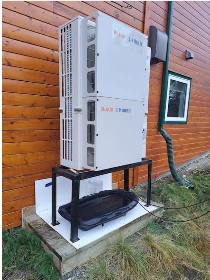
Figure 2: Outdoor unit of one participant showing wind baffles (to reduce ice buildup) and a sled used to periodically remove ice during the winter.
