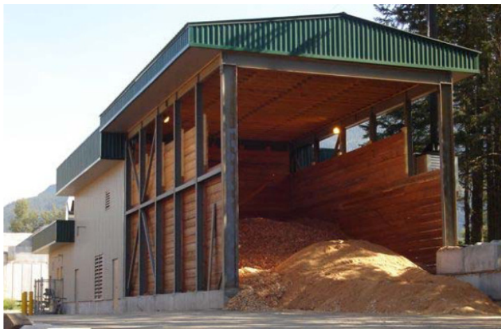
Figure 9: Biomass District Heating Plant in Revelstoke BC
