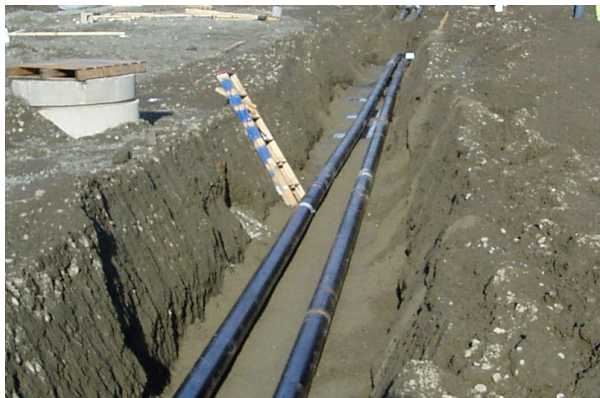
Figure 7: Example District Heating Distribution Pipe Installation
