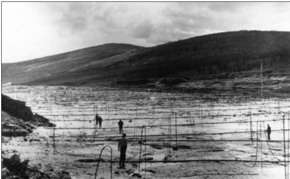
Steam points thawing ground in preparation for dredging. Klondike National Historic Sites/Willi Wandl Coll., neg. 445, serial #232
