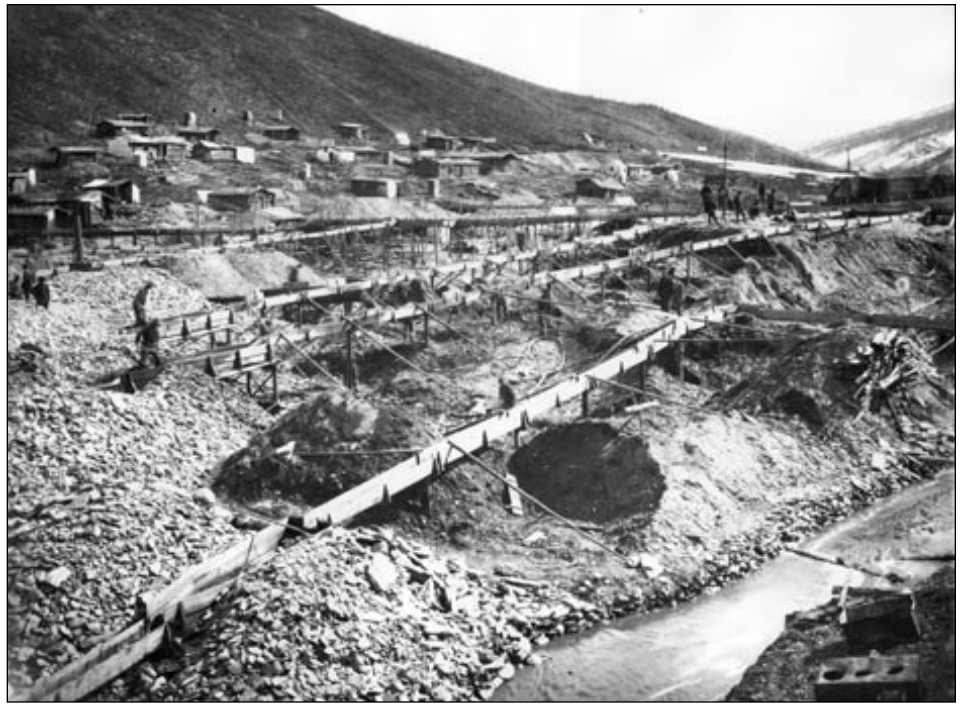
In the gold fields, flumes and sluicing go in every direction. Town of Eldorado, stores, a road-house and denuded hillsides in the background. Environment Canada, Parks, Headquarters, Anita Johns Coll., 116
