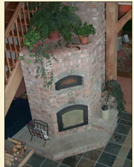
This Swedish masonry heater features a refractory cement core, secondary burning chamber, bake oven and 4.5-metre flame path. It adds heat to the home by acting like a huge radiator in the middle of an open concept house. Burns last for about two hours, consuming 23 kilograms of wood split to seven centimetres or less in diameter. The stove continues to provide heat to this 200-square-metre house for 12 or more hours, depending on the season, and uses only three to four cords of wood a year.
