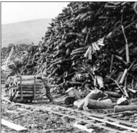
Huge piles of wood for steam thawing, 1912. Yukon Archives, Schellinger Coll, 6003
