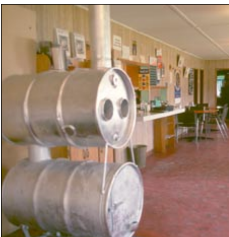
This woodstove, built by Phil Davignon, heated Johnson's Crossing Lodge even at -30^{\circ}\text{C} , using up to 40 cords of wood a year. Yukon government
