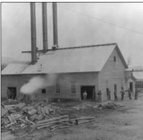
Power house at Bear Creek. Klondike National Historic Sites binder 42/167
