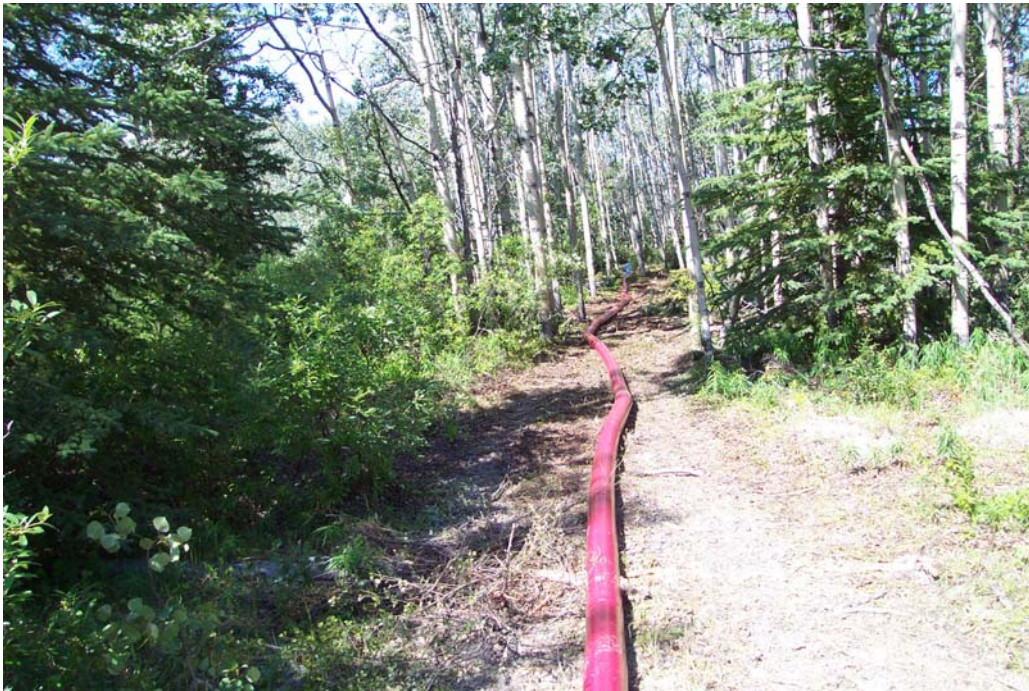
Photograph 3: Discharge line running northwest into wooded area, towards sewage outfall ditch.
