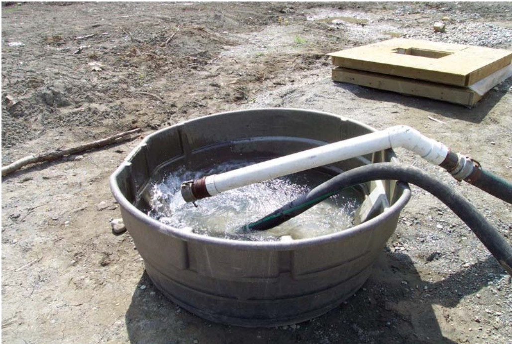
Photograph 5: Well flowing under Artesian pressure prior to beginning of pump test.
