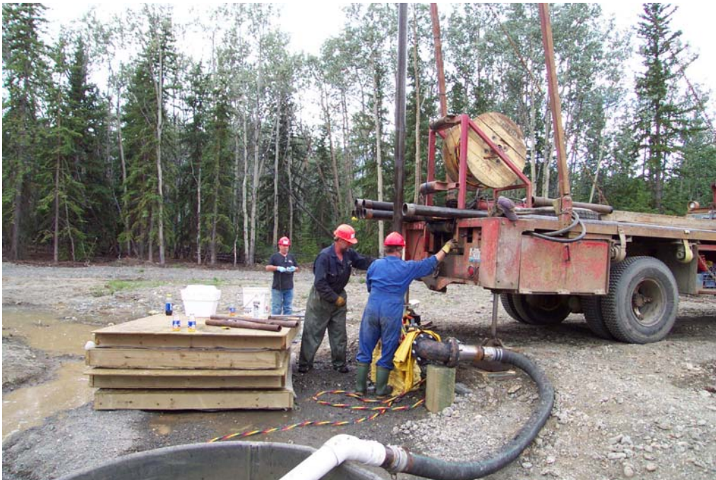
Photograph 9: Aqua Tech pulling pump and piping at termination of pump test
