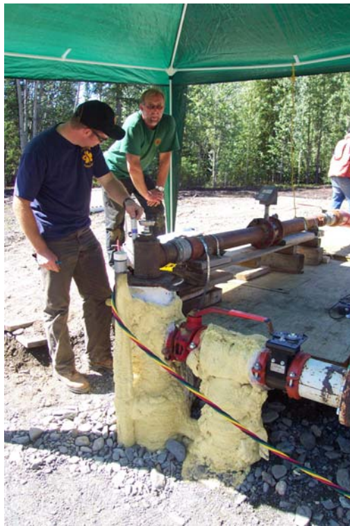
Photograph 7: Obtaining manual water level readings during pump test at Well 5.
