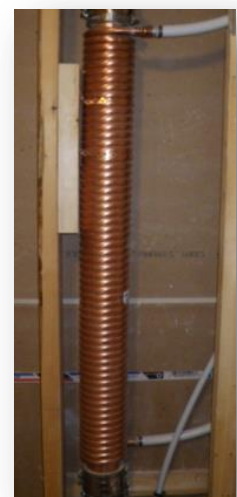
Figure 4: Drain water heat recovery
