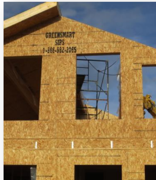
Figure 2: SIPs assembly
