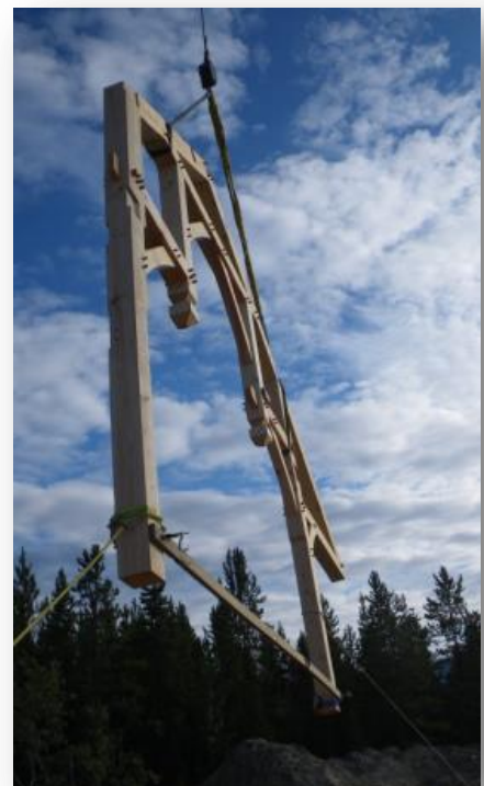
Figure 2: Setting timber structure
