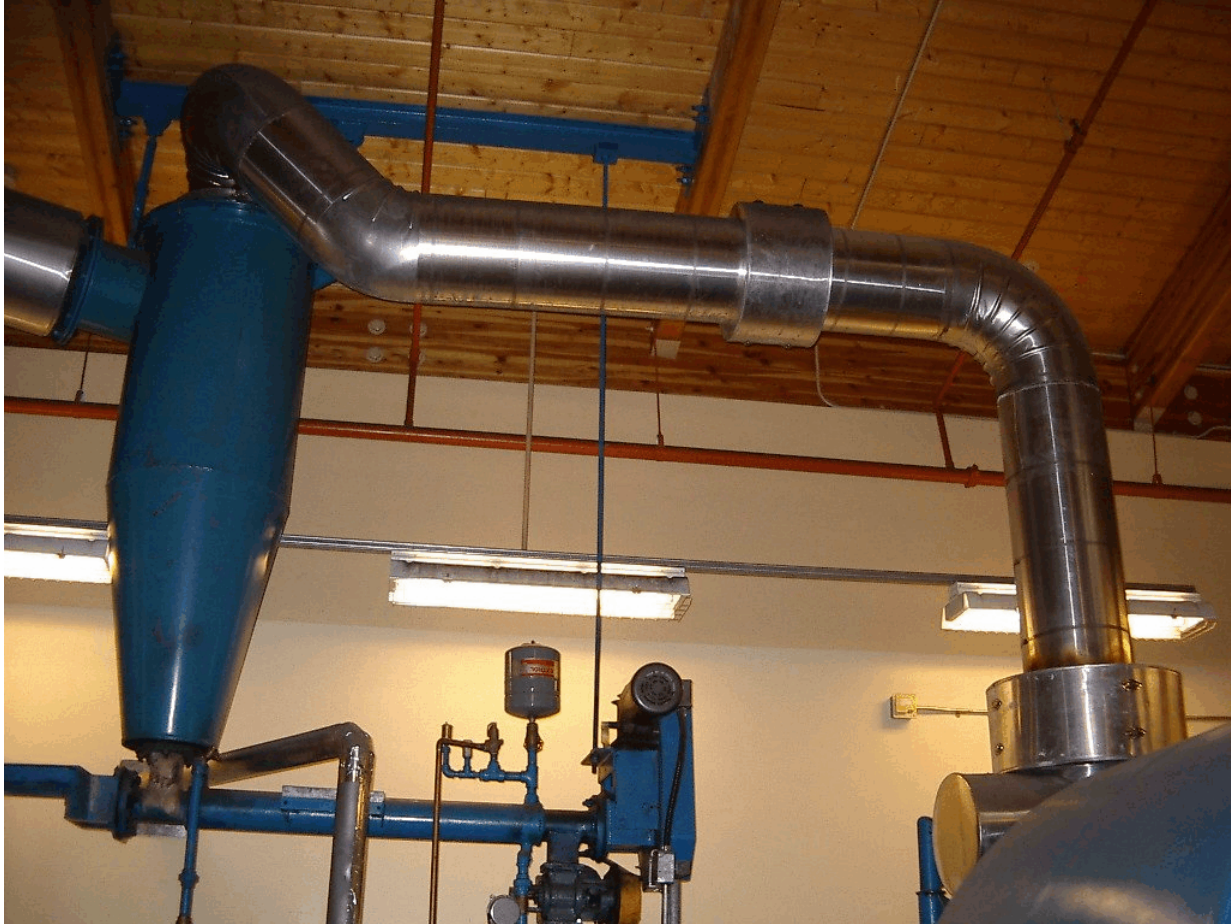
Figure 13. “Syngas” path from second cycle to boiler inlet
