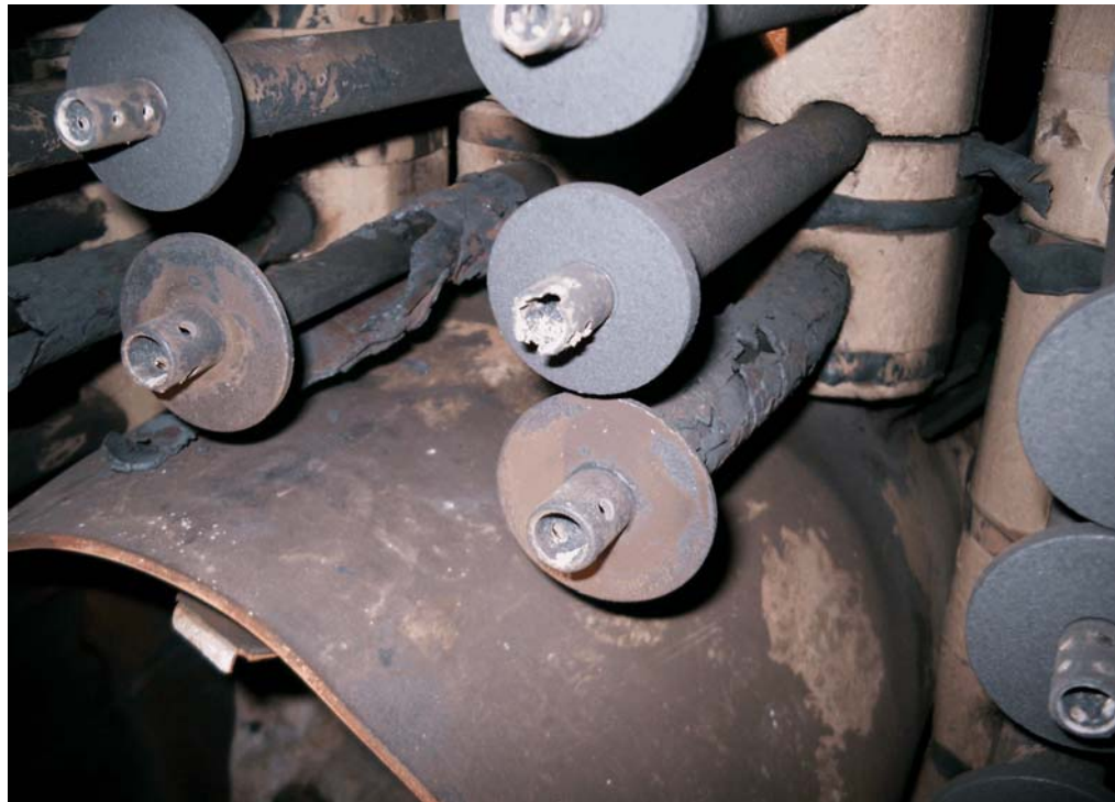
Figure 17. “Syngas” nozzles inside B1 Boiler
