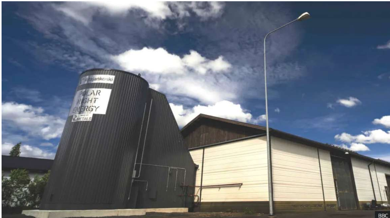
Figure 17: Sand-based TES at the Vatajankoski power plant in Kankaanpää, Finland [26]
