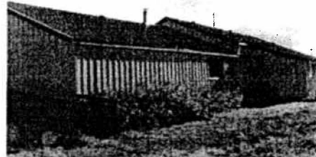
Figure 26 - Post Office/Bank/Library, Southwest Exposure
