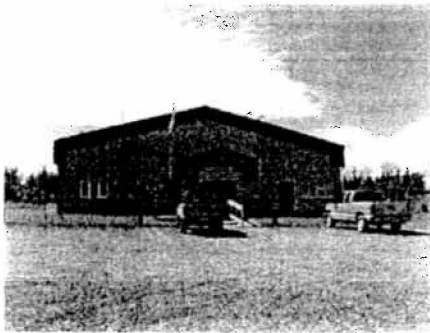
Figure 17 - Municipal Building, Eastern Exposure
