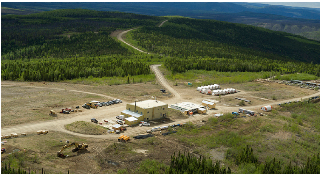
Brewery Creek Mine Infrastructure, source: Golden Predator Mining Corp. 130
