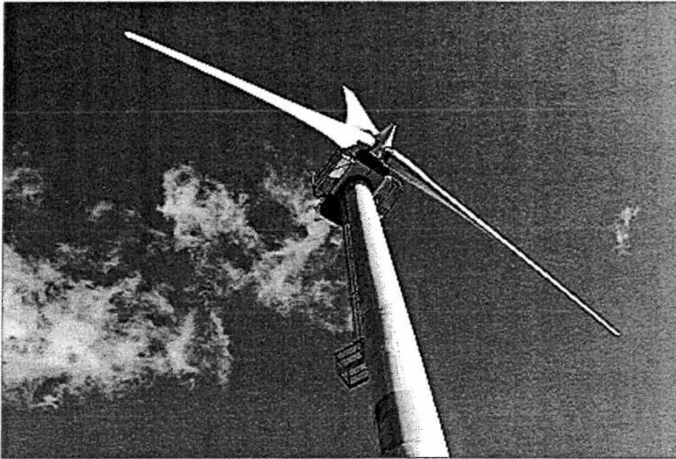
Wind turbine on Haeckel Hill in Whitehorse.
