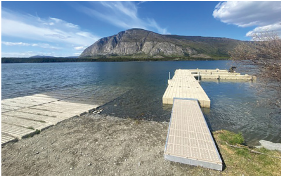
A new dock was installed at Pine Lake Campground.
