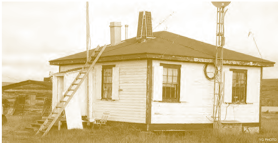
Royal Canadian Corps of Signals transmitter station - 1990.
