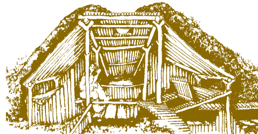
PRINCE OF WALES NORTHERN HERITAGE CENTRE, NT. (TERRANCE PAMPLIN)
