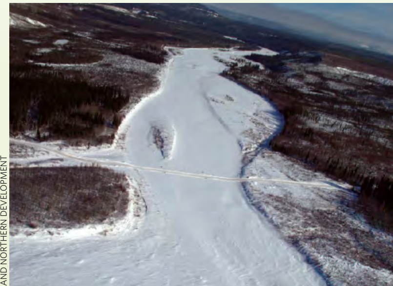
Ice bridge built over large stream channel
