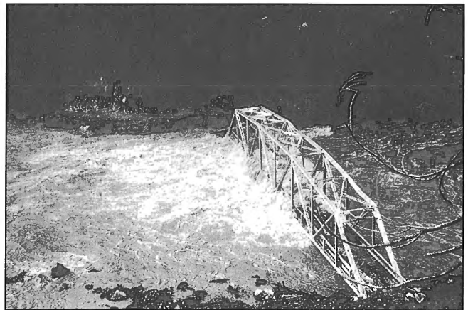
Figure 26. Jökulhlaup from Summit Lake, at Ninemile, Alaska, September 17, 1967. The discharge is almost 3000 \text{ m}^3/\text{s} , which is 100 times larger than the mean discharge of the stream at this site. The steel bridge was washed away a few hours after this photograph was taken. (Photo by J.J. Plummer).
