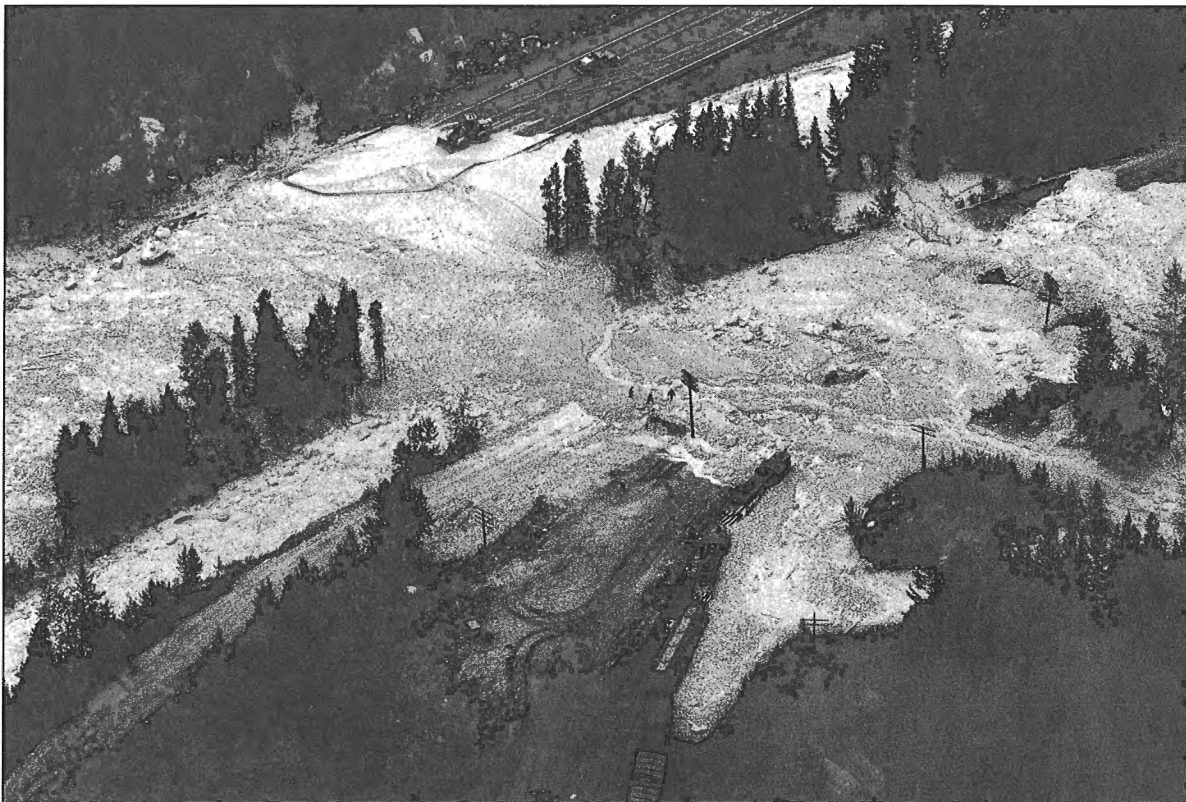
Figure 36. Debris flow deposits covering the Trans-Canada Highway and the Canadian Pacific Railway mainline in Kicking Horse River valley, September 7, 1978. Note the derailed and partially buried locomotives. (Photo by Calgary Herald, courtesy of Glenbow Archives, Calgary, Alberta).
