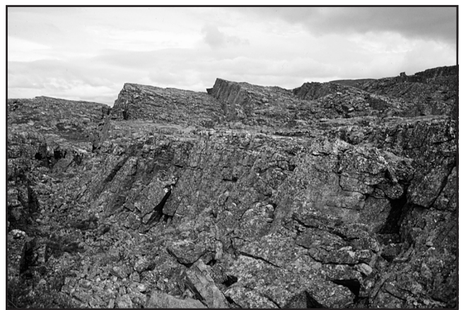
Figure 14. Rock-sag failure scarps (5 m high). Tonalite at junction of Soper and Livingstone rivers. Photograph by D.A. Hodgson. GSC 2001-379C
