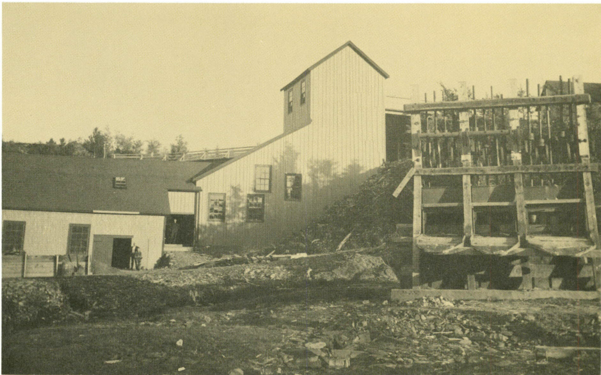
CRUSHER, CONCENTRATOR, AND REMAINS OF STAMP MILL, HALIFAX COUNTY, NOVA SCOTIA, 1891
