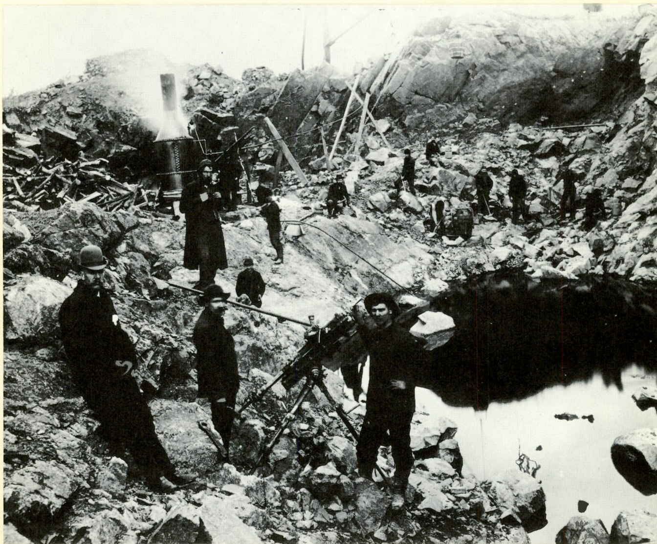
STEAM DRILLING AT SILVER LAKE MINE NEAR KINGSTON, ONTARIO, 1890
