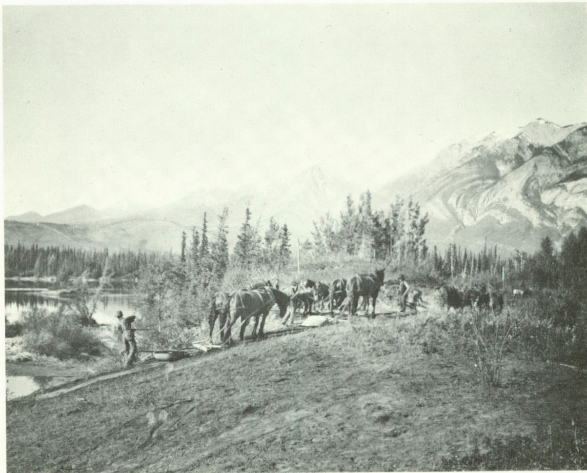
CONSTRUCTION WORK ON THE GRAND TRUNK PACIFIC RAILWAY IN WESTERN ALBERTA, 1910
