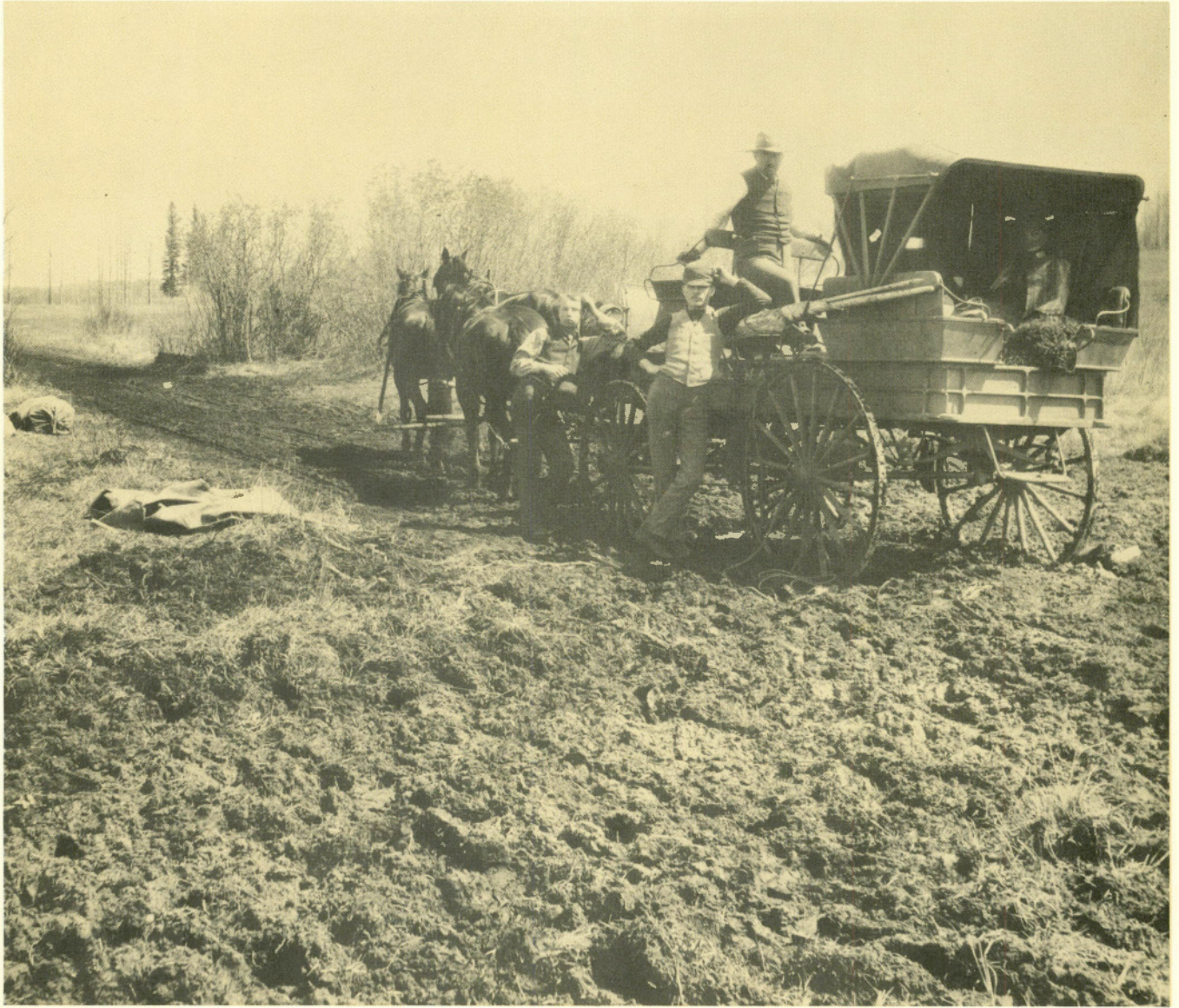
ROAD BETWEEN EDMONTON AND CALGARY, ALBERTA, 1889
