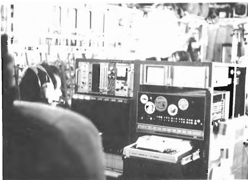
Figure 24.2 The GSC gamma-ray spectrometer installed in the Hercules CC-130 aircraft, was designed as a single self-contained unit on castor wheels and weighs over half a ton. The MRS navigational units (see text) were conveniently mounted on one end of the spectrometer for operation by a military navigator.
