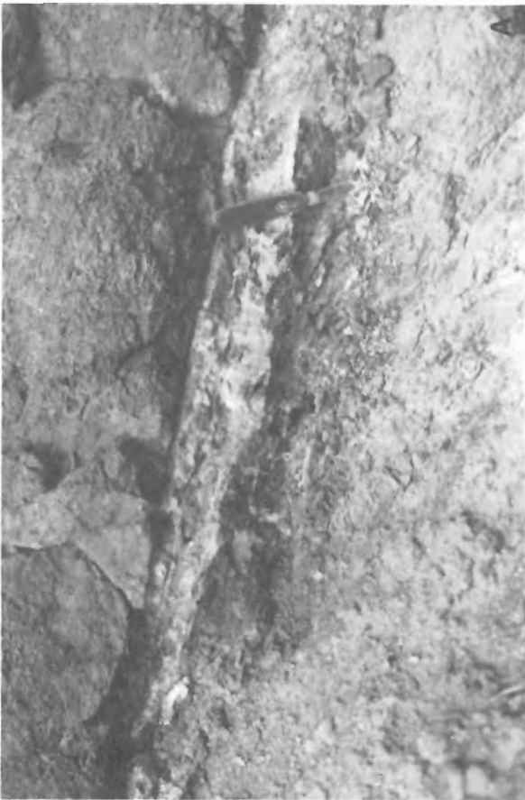
Figure 4.a. Clay zone developed along bedding plane in upper tuff zone; slickensides are found at clay/tuff interface.
