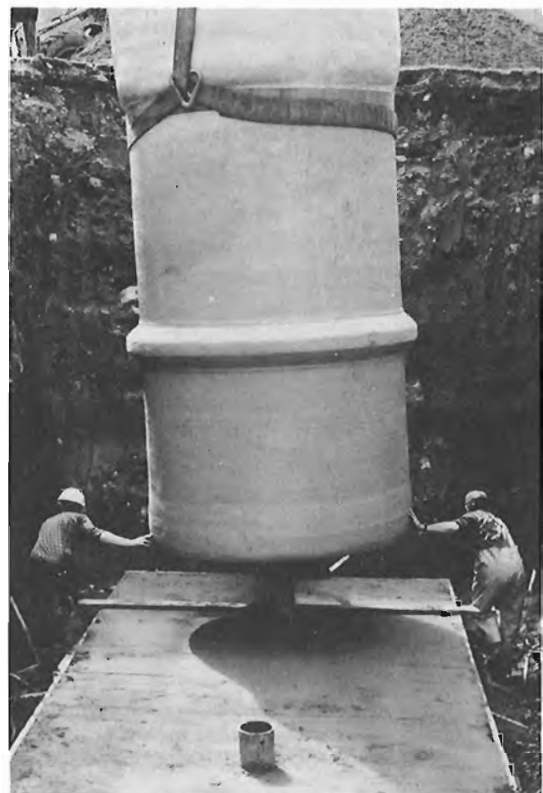
Figure 3.23. Positioning the fiberglass tank in the excavation at the Nova Scotia Research Foundation Corporation. The run pipe for the second tank can be seen in the foreground protruding through the concrete base. The hole in the bottom of the tank is positioned over the run pipe. After installation it is attached to the tank with a watertight fiberglass bond. (GSC 203256-W.)
