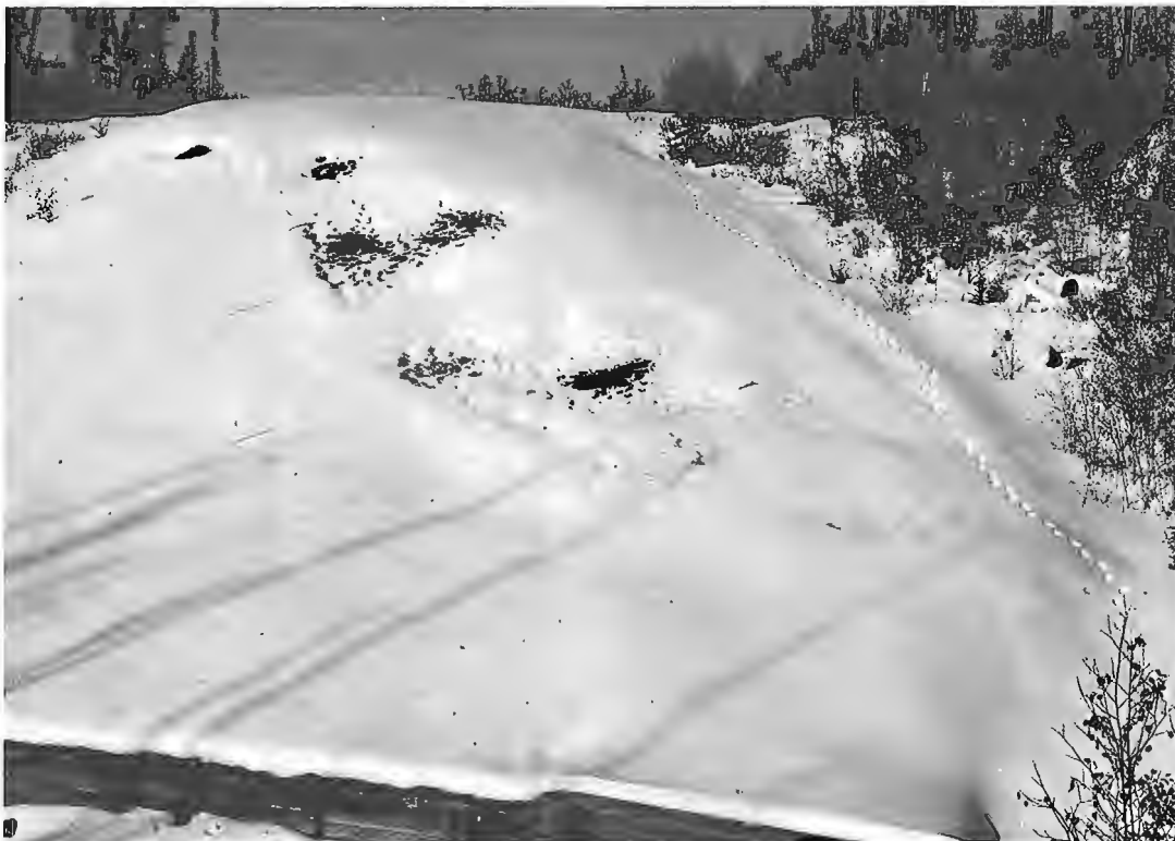
Figure 8. Hot spots, slope 44, October 1992. Extensive snow melt across right-of-way.
