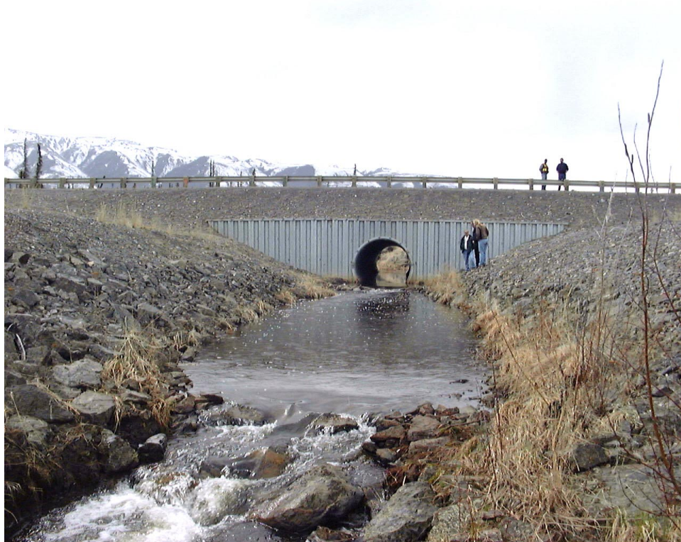
Swede Johnson Ck. multiplate with fish weir, Feature DB027
