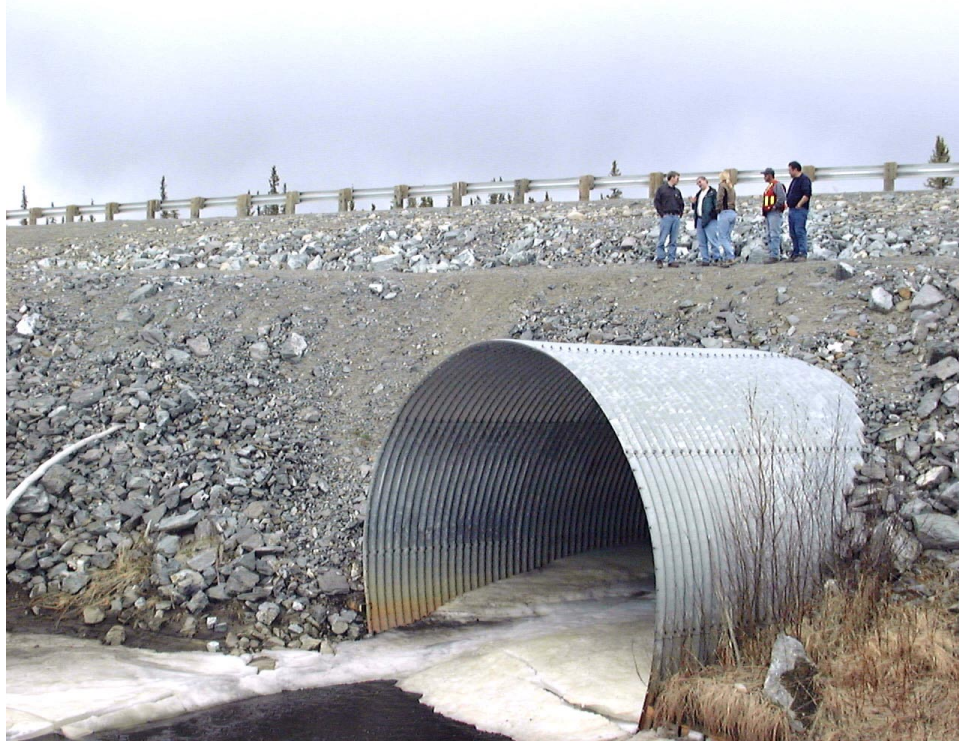
Longs Creek culvert, Feature BC044
