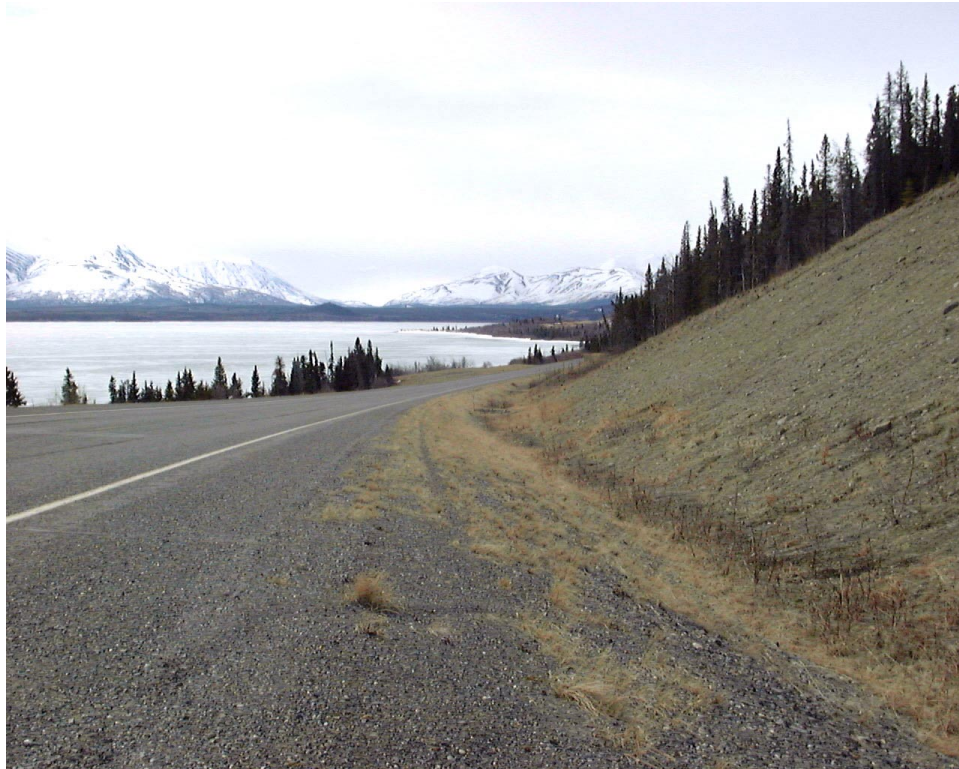
129 Hill, showing ditch blocking, Feature HJ007
