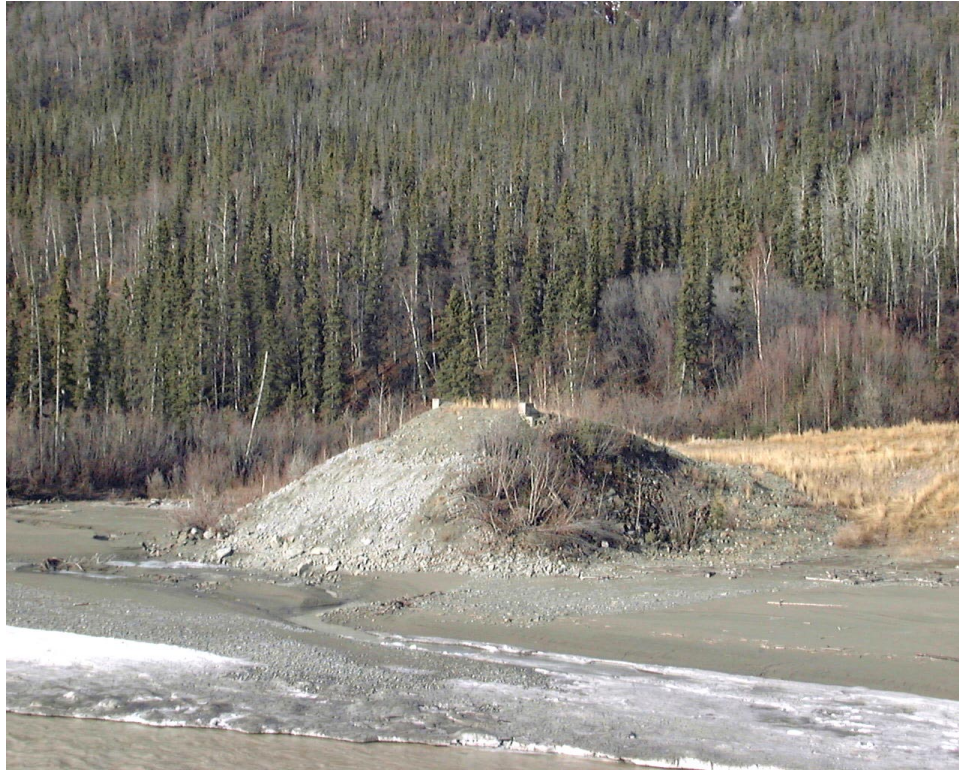
Old bridge abutment at White River, Feature BC075
