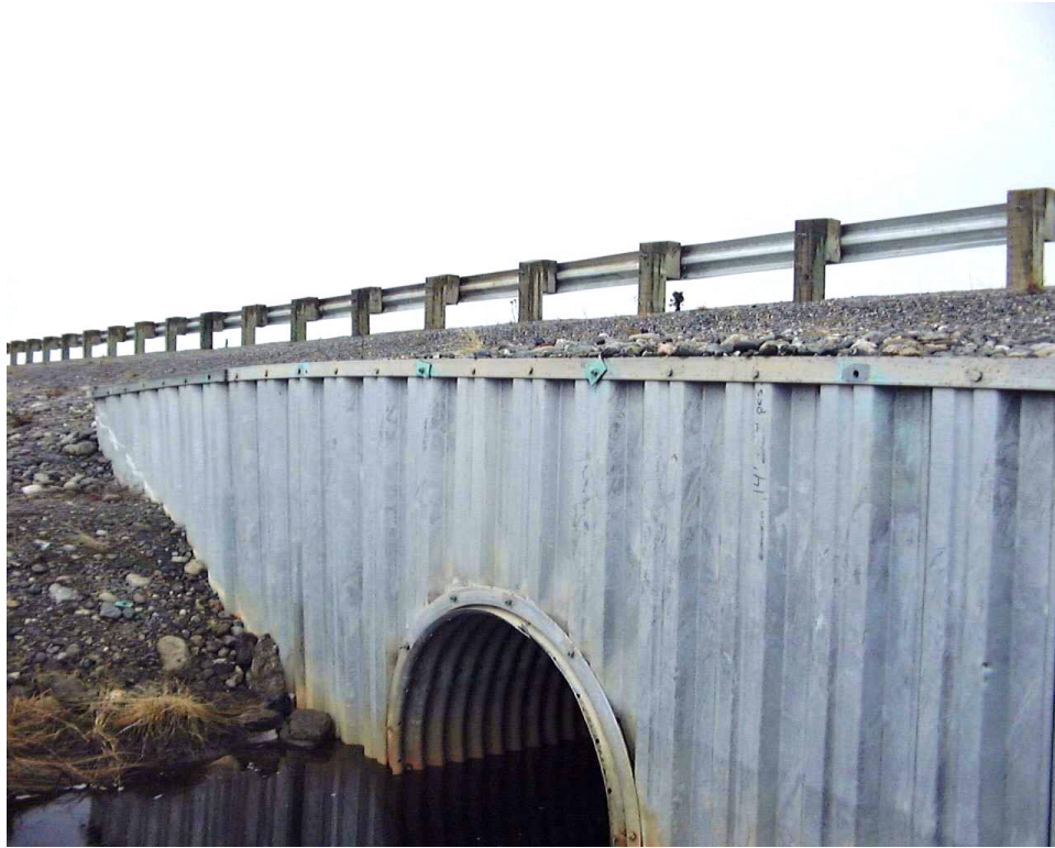
Multiplate - Enger Creek, Feature BC143
