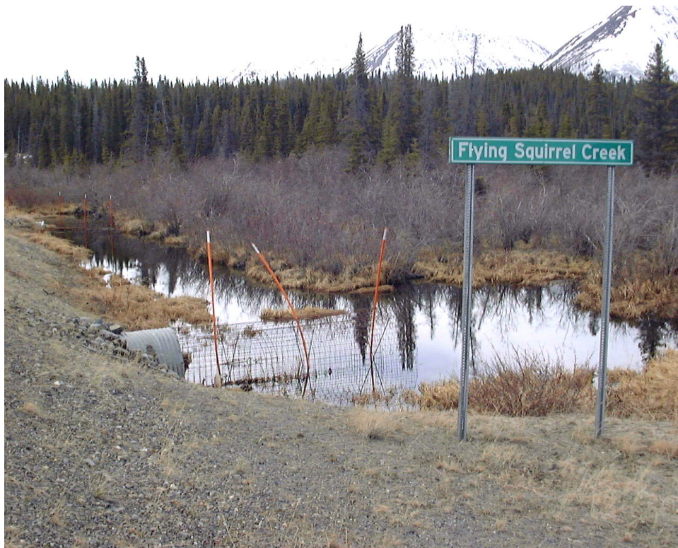
Culvert at Flying Squirrel Creek, showing beaver deterrent structure, Feature BR168
