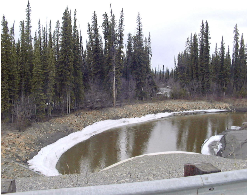
Snag Creek, showing armoured bank, Feature BC167
