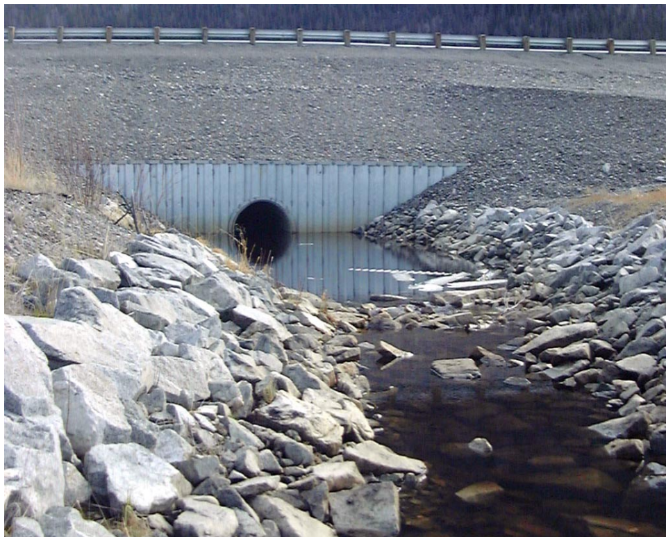
Icing Culvert with rock weir, Feature BC037
