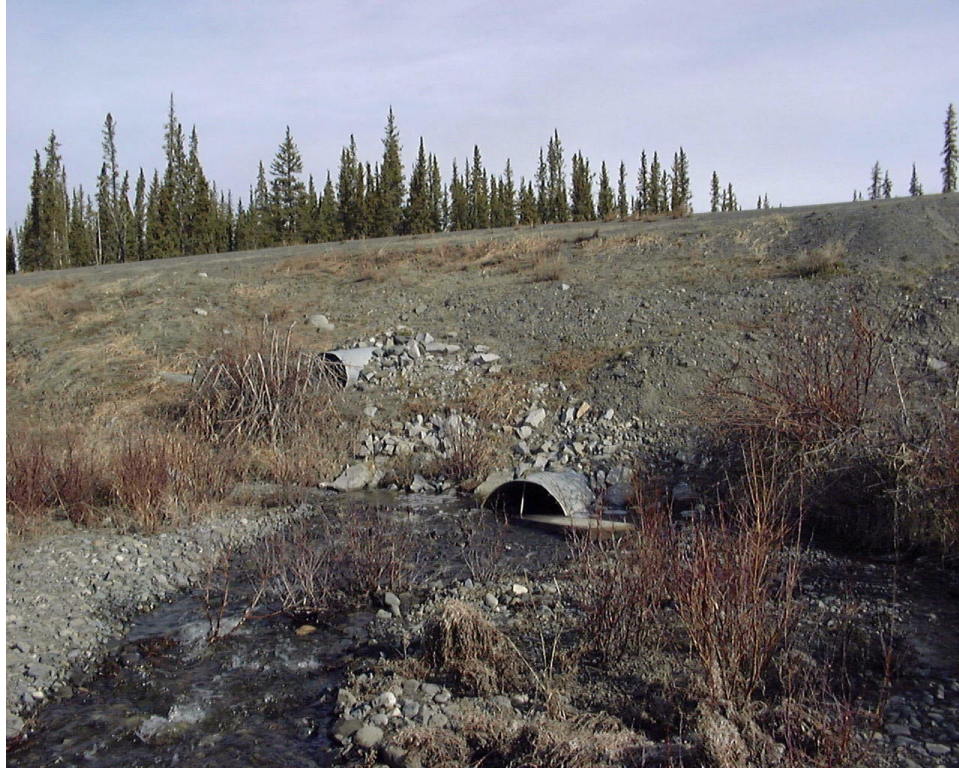
Icing Culvert, Feature HJ047
