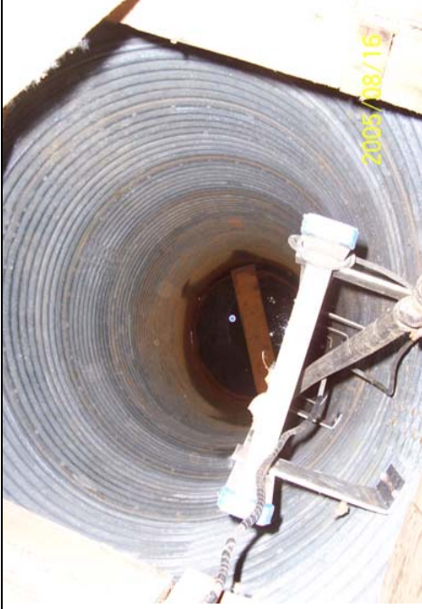
Photo 003: Looking down abandoned dug well.
