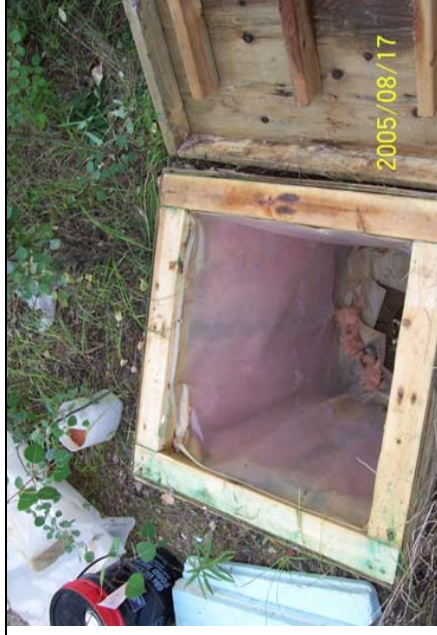
Photo 056: 5650 Wellhead enclosure.
