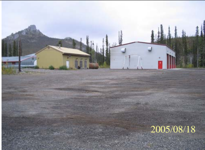
Photo 206: 2661 Olgilvie grader station.
