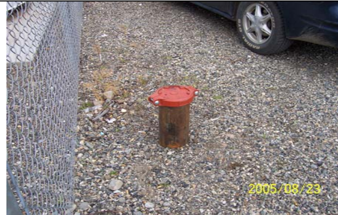
Photo 399: 5676 Monitoring well for rock pit drain.
