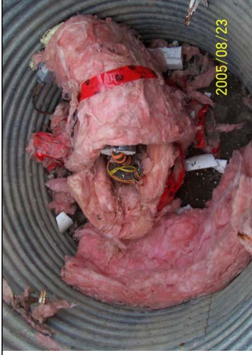
Photo 394: 5987 Well enclosure and wellhead in pit.
