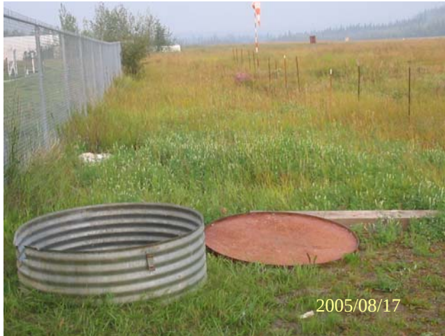
Photo 0187: 5653 Mayo Airport wellhead enclosure.
