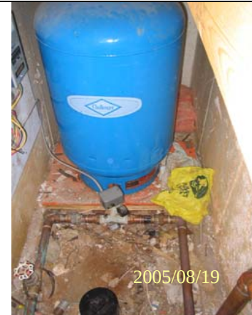
Photo 234: 2544 Abandoned well (bottom) pressure tank & pump controls (top).
