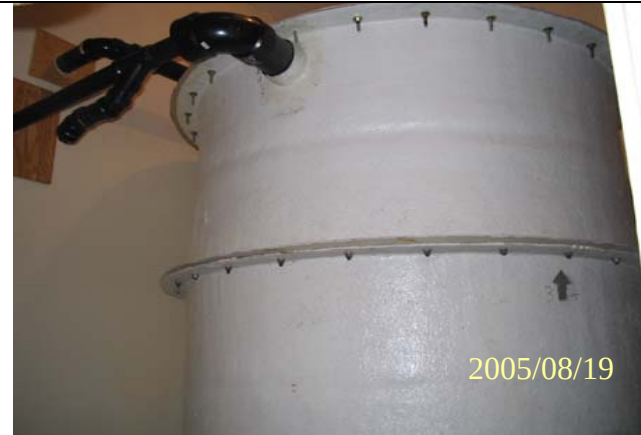
Photo 225: 2575 Water storage tank.
