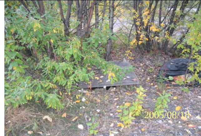
Photo 213: 2665 On site sewage disposal for grader station.
