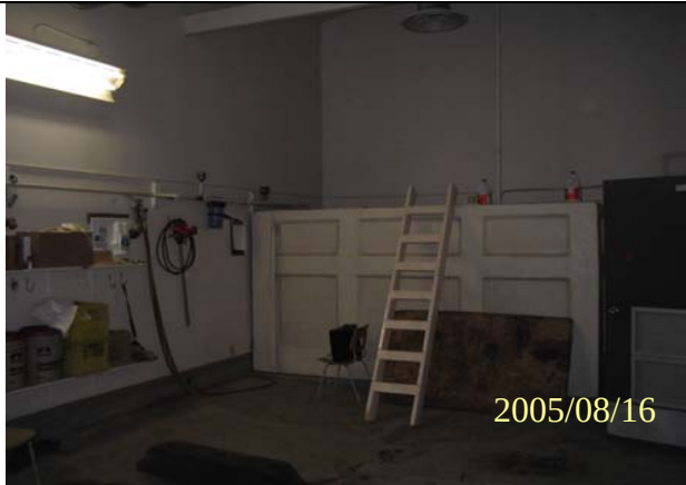
Photo 179: 5622 Main water storage tank.
