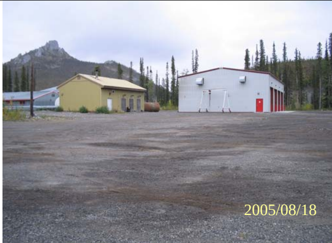
Photo 206: 2661 Olgilvie grader station.
