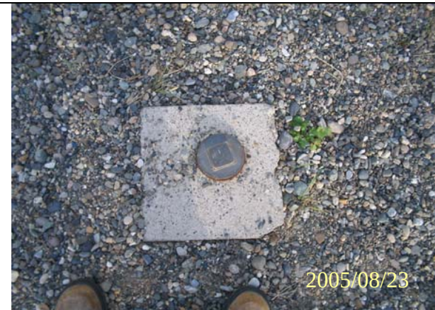
Photo 214: 5672 Potential septic clean out?
