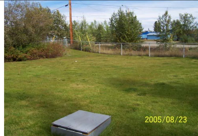
Photo 381: M0156/M0226 Well enclosure.
