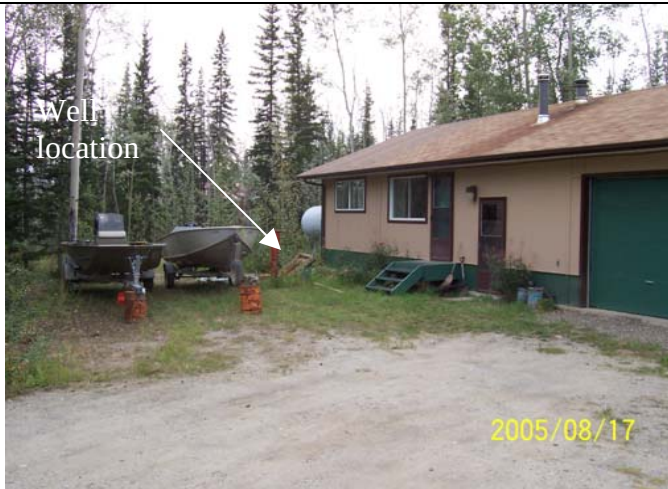
Photo 033: 5650 Wildlife Workshop (northeast side of building).
