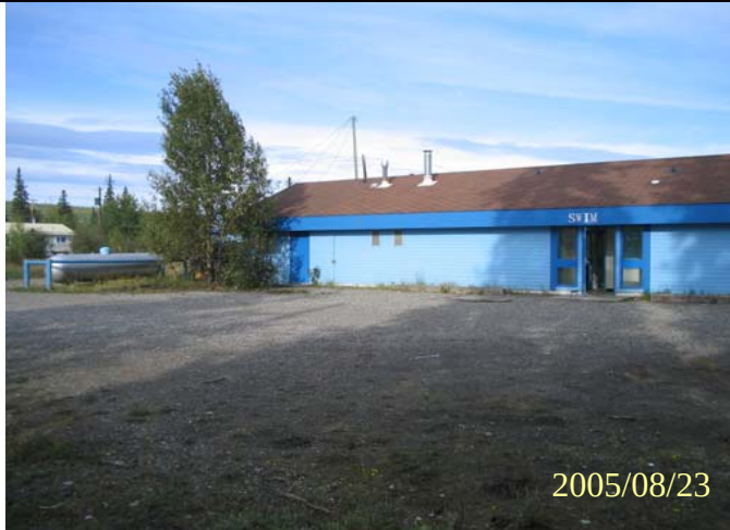
Photo 209: 5672 Pelly Crossing swimming pool. (northeast)
