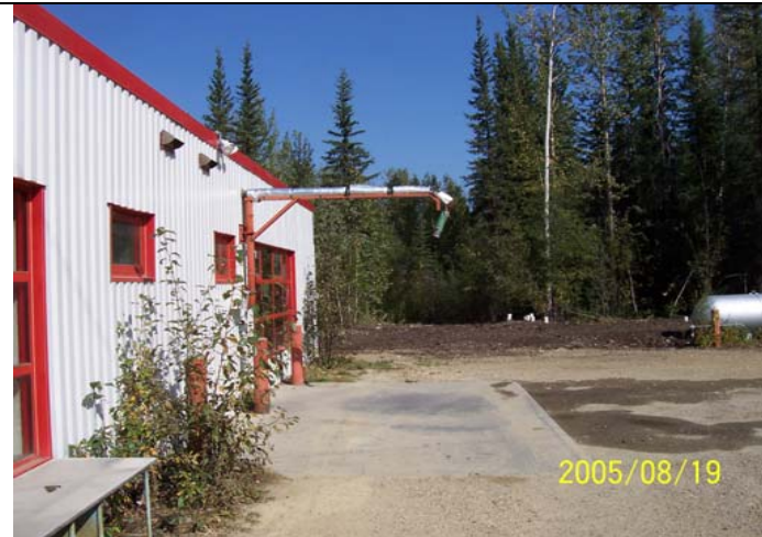
Photo 096: 2592 Water filling station.
