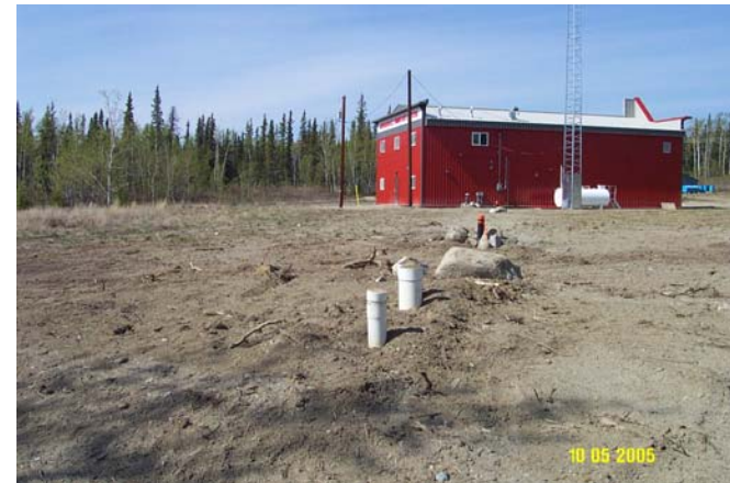
Photo 0094: 1421 Septic Field (front) and Mendenhall Firehall (back)
