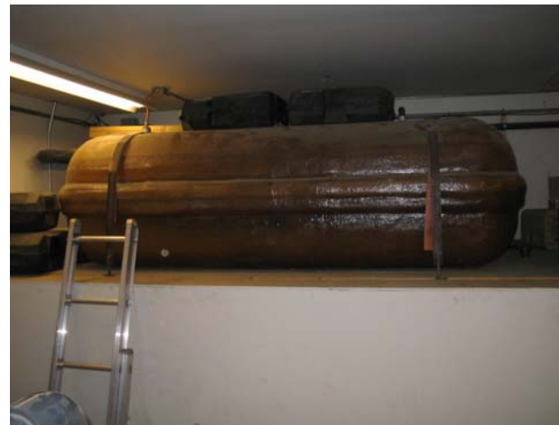
Photo 0470: 1924 Water Storage Tank
