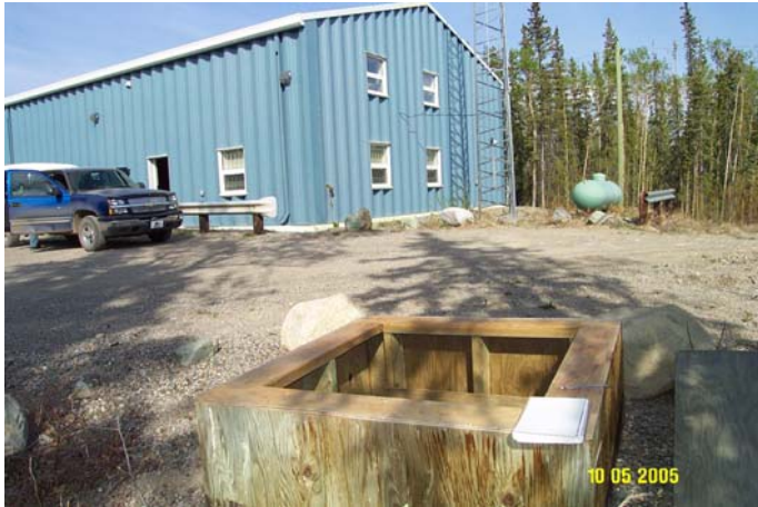
Photo 0100: 1950 Well-Enclosure – Pit (front), Ibex Valley Firehall (back)
