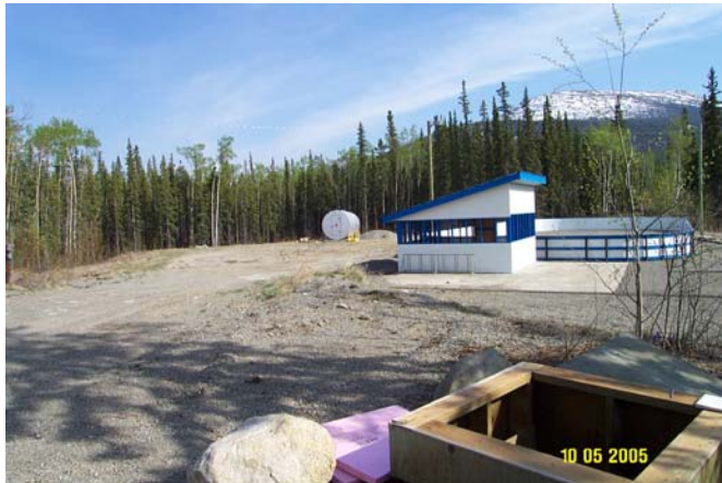
Photo 0101: 1950 Well (front), Skating Rink and Above Ground Oil Storage Tank (back)
