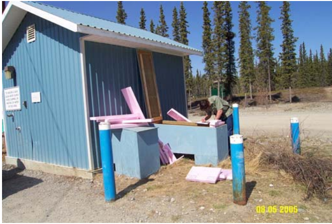
Photo 0062: 1953 Well Enclosure (right) and Pumphouse
