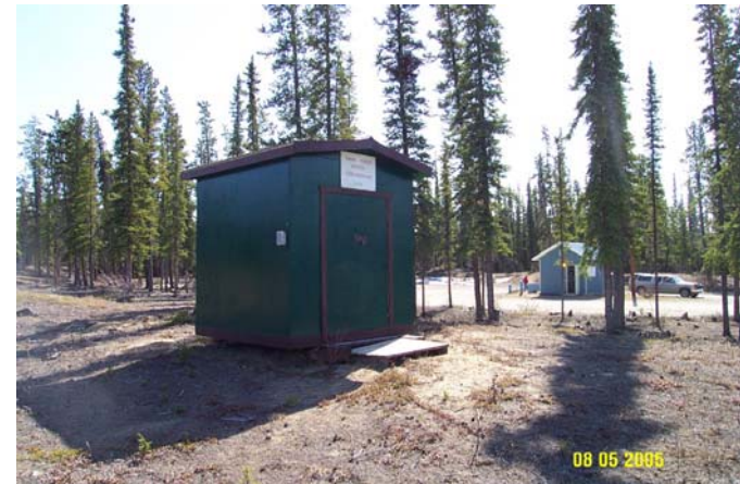
Photo 0060: 1953 Fire Equipment Cache (front), Pumphouse (back left)
