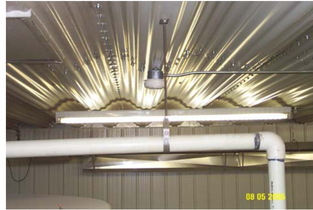
Photo 0067: 1953 Pipe Hangar – Potential Location for Solenoid
