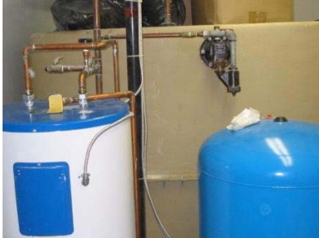
Photo 0018: 1955 Hot Water Tank (left) and Pressure Tank (right)
