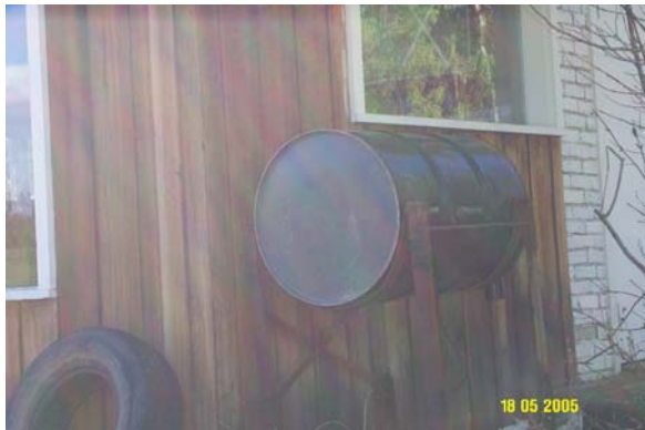
Photo 0182: YWP-B Above Ground Fuel Storage Tank
