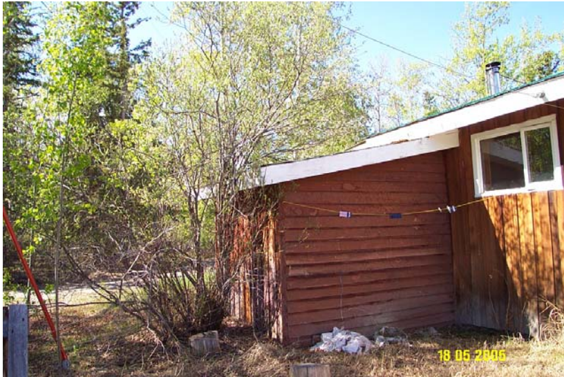
Photo 0183: YWP-B Preserve Staff Building and Well House Addition
