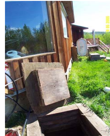
Photo 0178: YWP-A Well Head Enclosure (front), Main Office (left) and Above ground Fuel Storage Tank (right)
