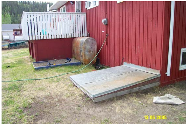
Photo 0166: M0201 Wellhead (front below paneling), R.C.M.P. Residence (behind) and Above Ground Storage Tank (center)
