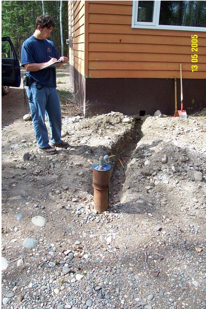
Photo 0163: 6536 Wellhead (front) and Forestry Crew Quarters (back)
