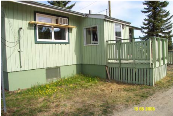
Photo 0155: 6542 Forestry District Office (wellhead located inside underneath)
