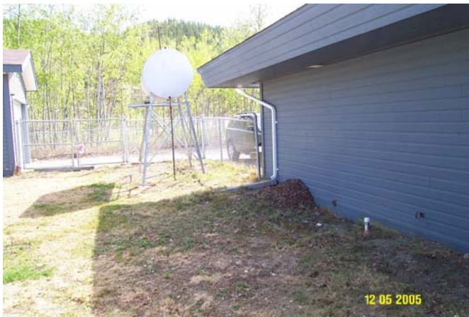
Photo 0138: 6975 Above Ground Fuel Storage Tank and Hydrocarbon Spill Site
