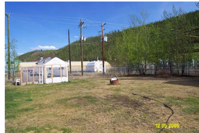
Photo 0139: Substation and Above Ground Fuel Storage Tank (back)
