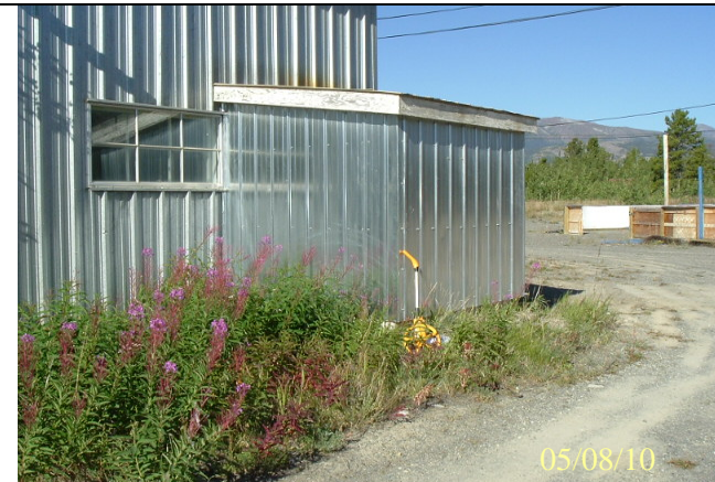
Photo 028: 1131 Abandoned wellhead enclosure.
