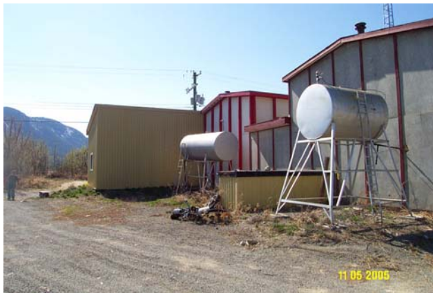
Photo 0124: 1137 Above Ground Storage Tanks Adjacent to Well
