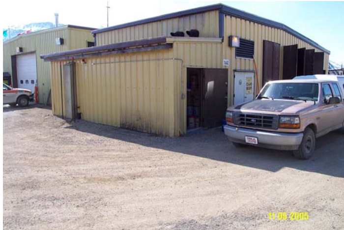
Photo 0111: 1500 Maintenance Garage with access to Water Equipment Room
