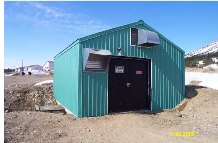
Photo 0112: 1500 Hydroelectric Generating and Penstock Station
