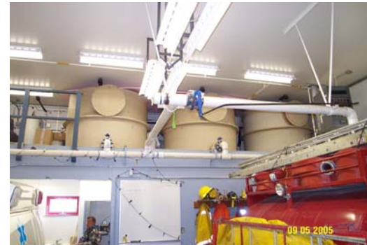
Photo 0074: 1334 Tanks and Truck Fill (domestic tank far right)
