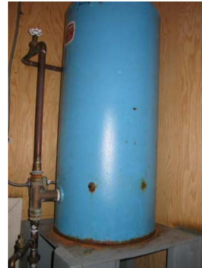
Photo 0022: 6542 Pressure Tank
