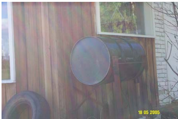
Photo 0182: YWP-B Above Ground Fuel Storage Tank
