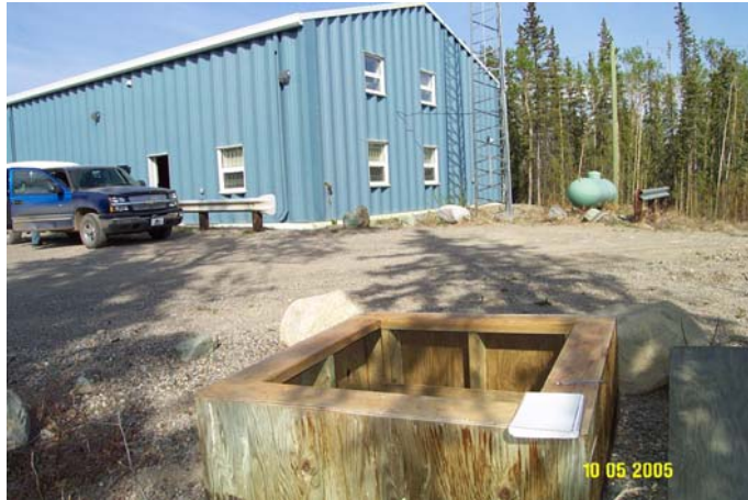
Photo 0100: 1950 Well-Enclosure – Pit (front), Ibex Valley Firehall (back)
