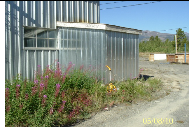
Photo 028: 1131 Abandoned wellhead enclosure.
