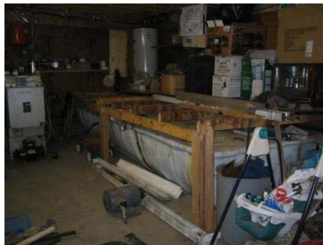
Photo 0006: YWP-D Water Storage Tank
