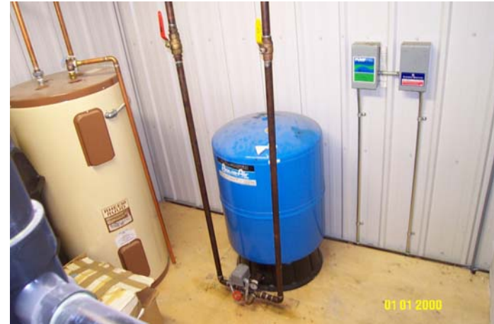
Photo 0106: 1950 Pressure Tank
