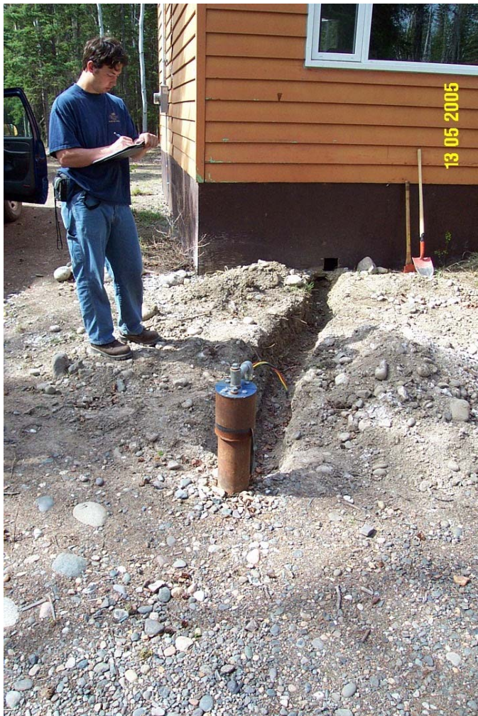
Photo 0163: 6536 Wellhead (front) and Forestry Crew Quarters (back)
