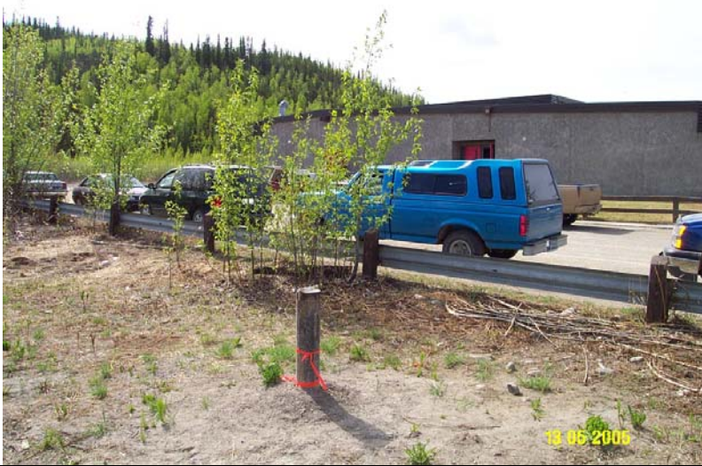
Photo 0159: 6511-C New Well Wellhead
