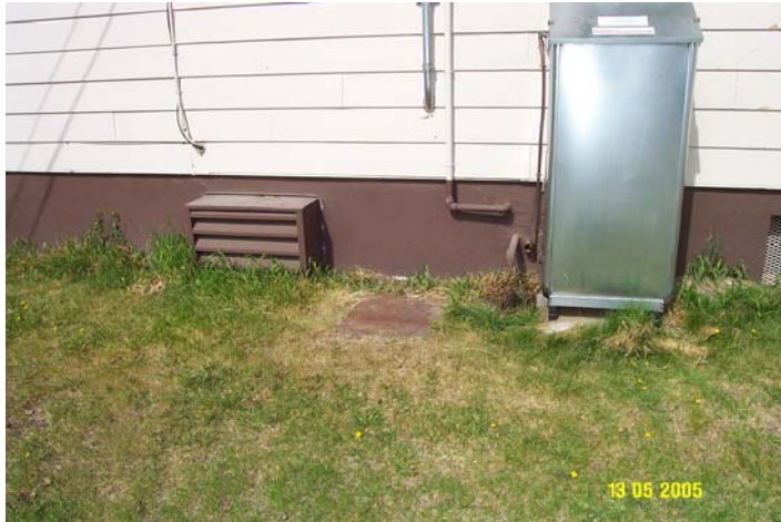
Photo 0162: 6511-A Main School Wellhead (underneath panel at center) and Above Ground Fuel Storage Tank (right)
