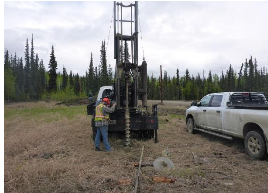
Auger drilling borehole BH 5-18
