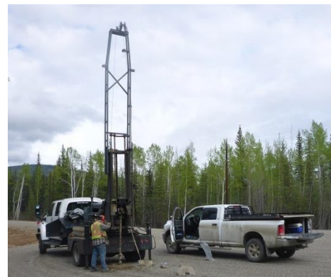
Drilling of borehole BH 6-18
