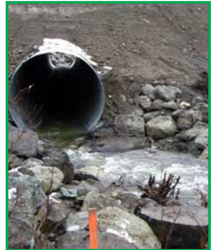
Closed bottom culvert. The culvert must be angled to allow water to flow freely through the culvert.
