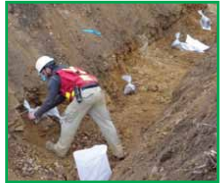
The sides of trenches should be sloped to a stable, safe angle to limit the safety risk associated with entrapment from slumping.
