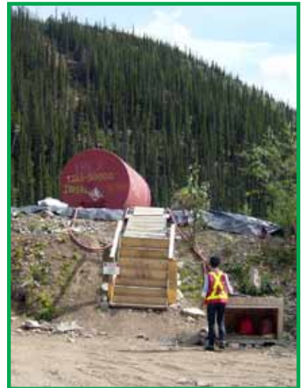
Stationary fuel containers with secondary containment. Note earth berm lined with plastic and signage posted at foot of stairs and on the fuel tanks.
