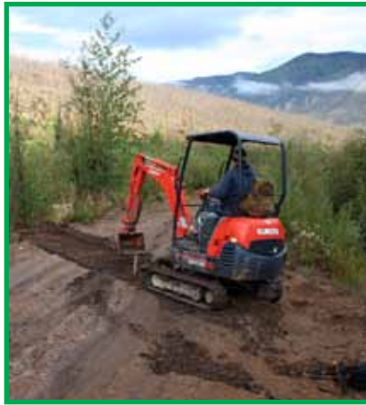
Construction of a water bar to divert surface runoff. Water bars should be constructed at an angle and in the fall to help divert spring runoff.
