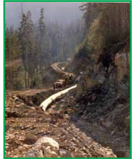
Ditches and culverts should be designed not to discharge water directly into watercourses or onto erosion prone slopes. Note the ditch is “u” shaped.
