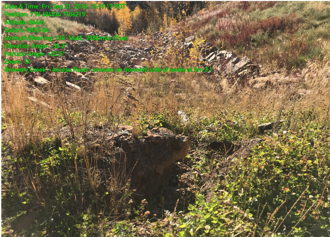
Photo 7: Riprap drainage swale No. 2 at about km 2.9 (recorded as km 3.1 in the field), looking downslope from edge of road. Note minor erosion in the foreground.
