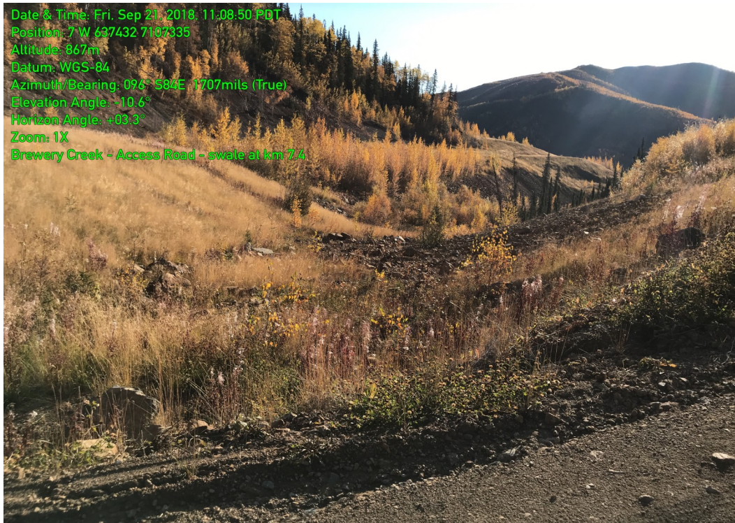
Photo 10: Drainage swale No. 6 at about km 7.4, looking downslope from road surface. Water ponds on uphill side and discharges from toe of rip rap about 100 m downslope, in approximately the centre of the frame.
