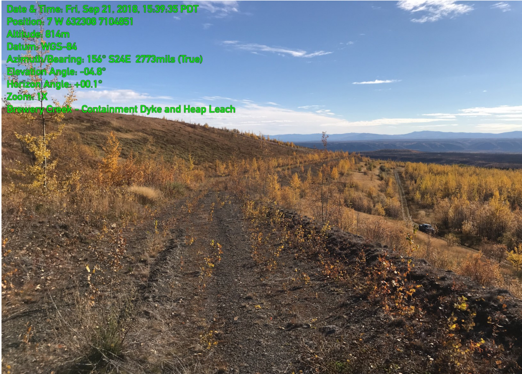
Photo 19: Heap leach and containment dyke (from crest of dyke).
