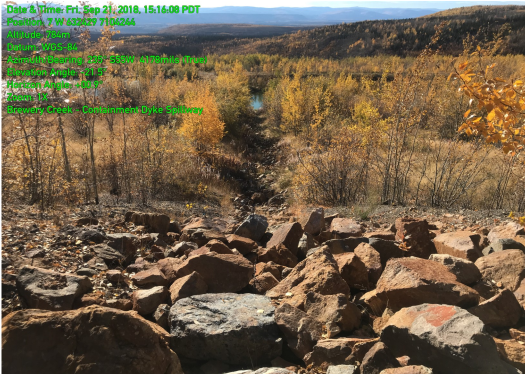
Photo 20: Heap leach spillway.
