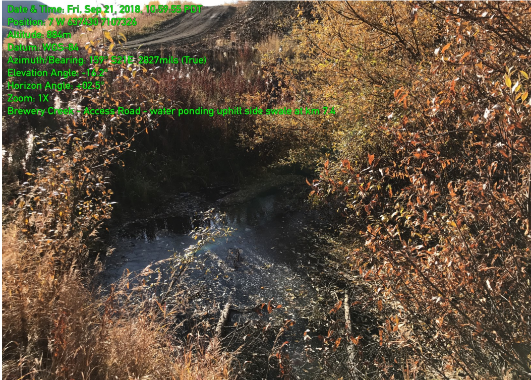
Photo 9: Water ponding against uphill side of the road at drainage crossing No. 6 at about km 7.4. No culvert or other means of drainage across the road was visible.
