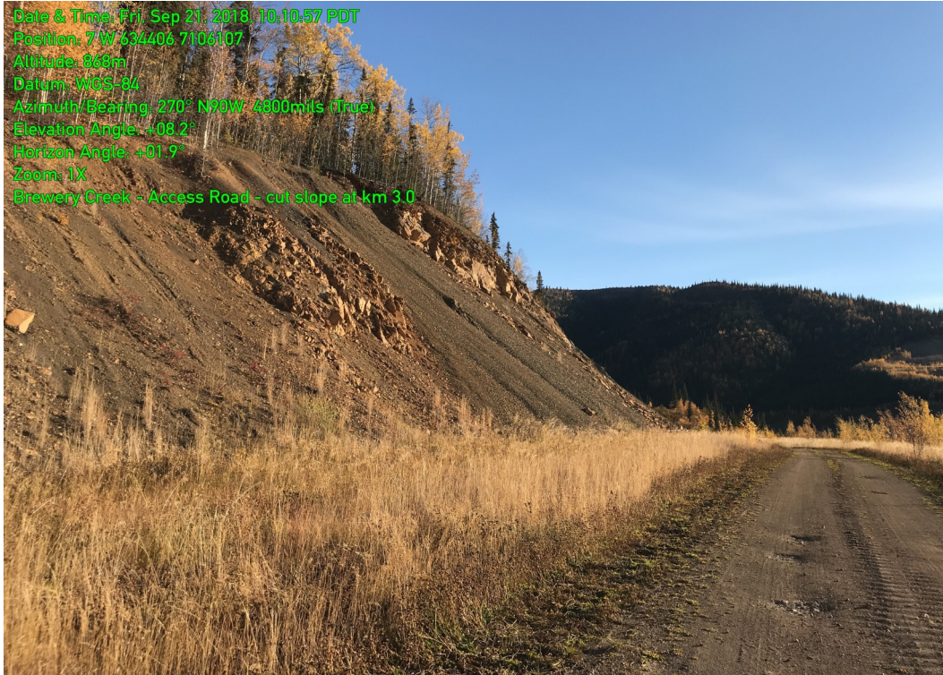
Photo 5: Cut slope at about km 3.0.
