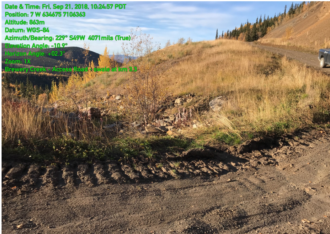
Photo 8: Riprap drainage swale No. 3 at about km 3.3. Note minor erosion gully developed by water flowing across and off the downslope side of the road.
