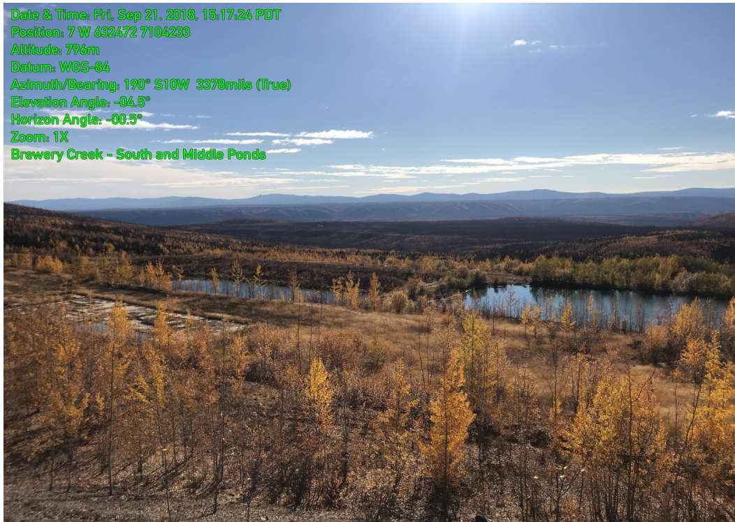
Photo 26: South and Middle Ponds viewed from crest of containment dyke. Note high water in middle pond and very low water in south pond.
