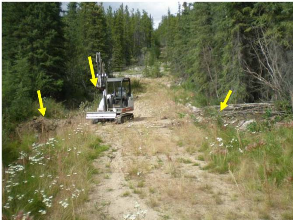
Photograph 13: Yellow areas show where diversion ditches were excavated to redirect surface water runoff from the road side into the vegetated areas on either side of the access road.
