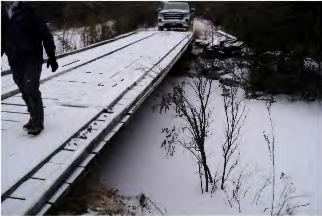
Photograph 17: Bridge Crossing at Merrice Creek – Upstream Side
