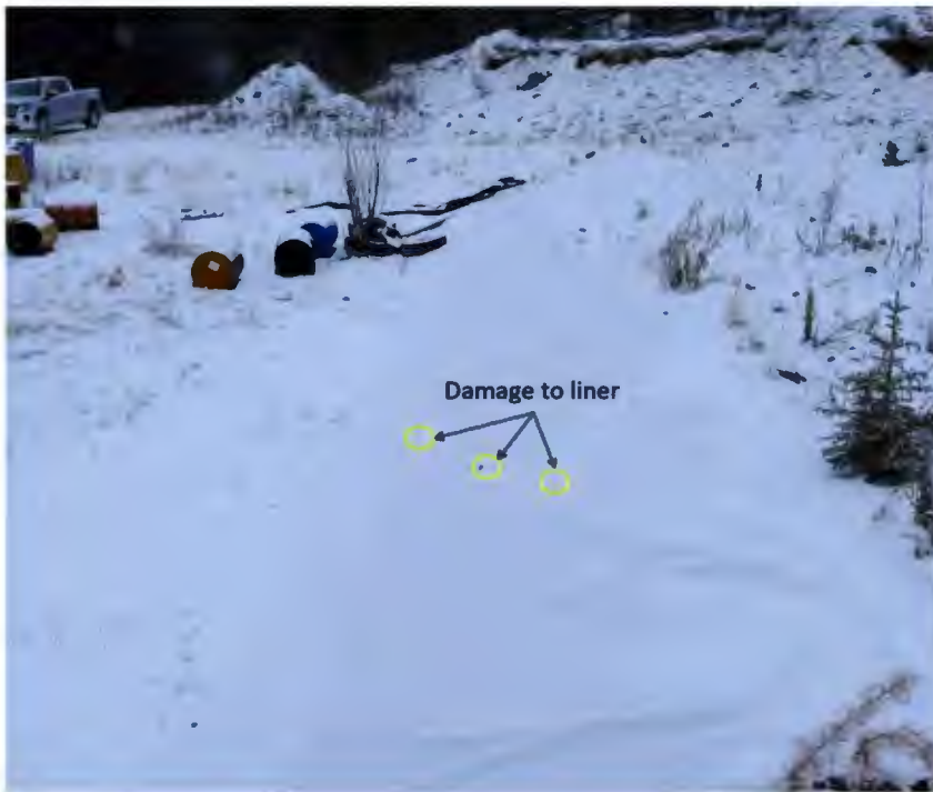
Photograph 11: Liner Damage at Fuel Storage Area
