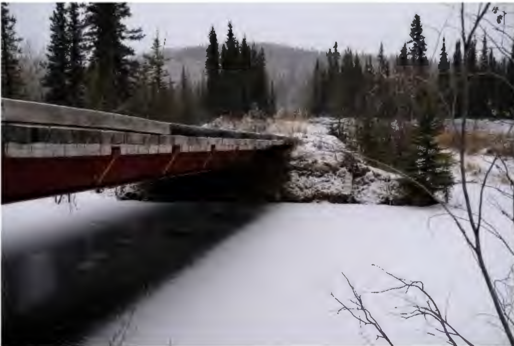
Photograph 16: Bridge Crossing at Merrice Creek – Downstream Side
