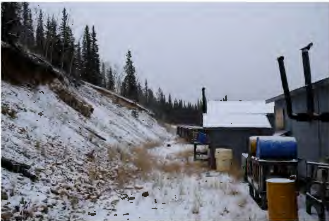
Photograph 4: Cut-slope behind the Camp Geology Office and Core Logging Shack
