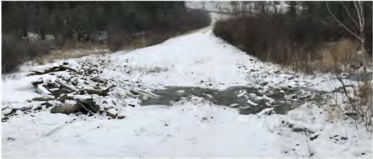
Photograph 15: Williams Creek Ford Crossing
