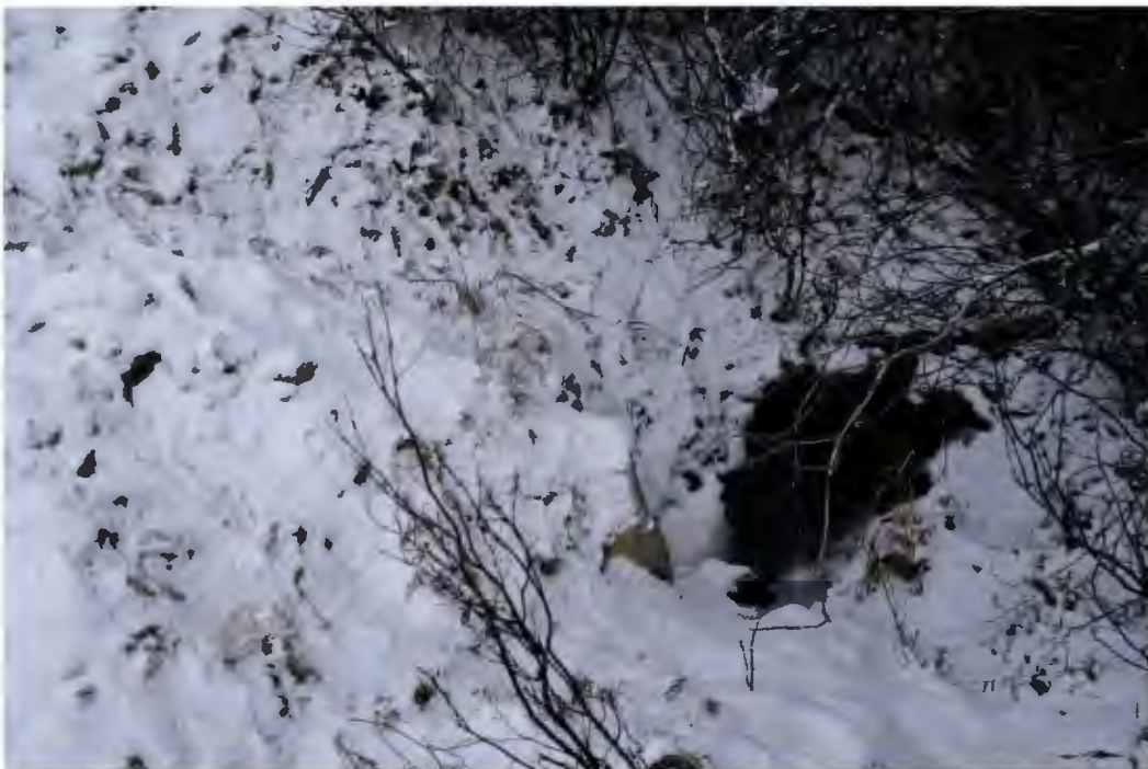
Photograph 14: Culvert Outlet beneath Road at North Williams Creek
