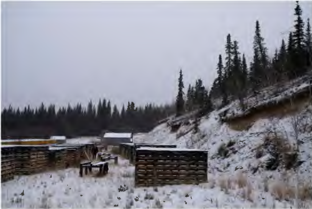
Photograph 3: Cut-slope behind Camp Geology Office and Core Shack
